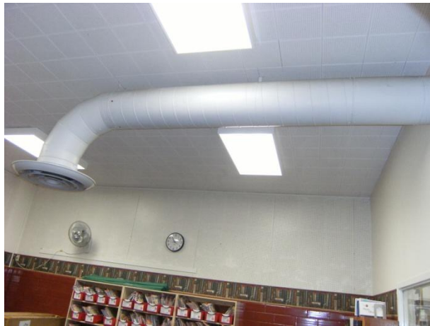
Figure 8: Reference Room Branch Duct
