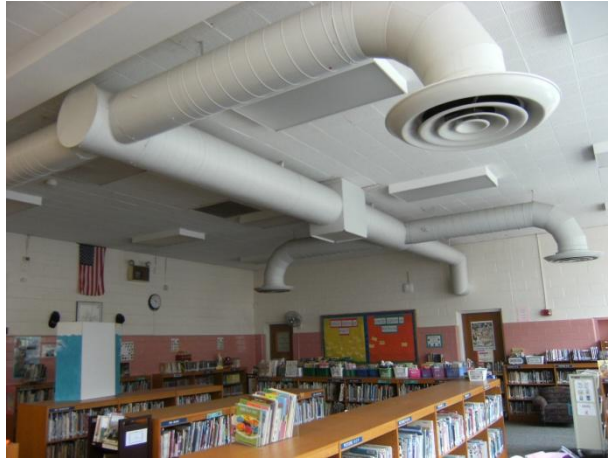
Figure 7: Library Duct Distribution
