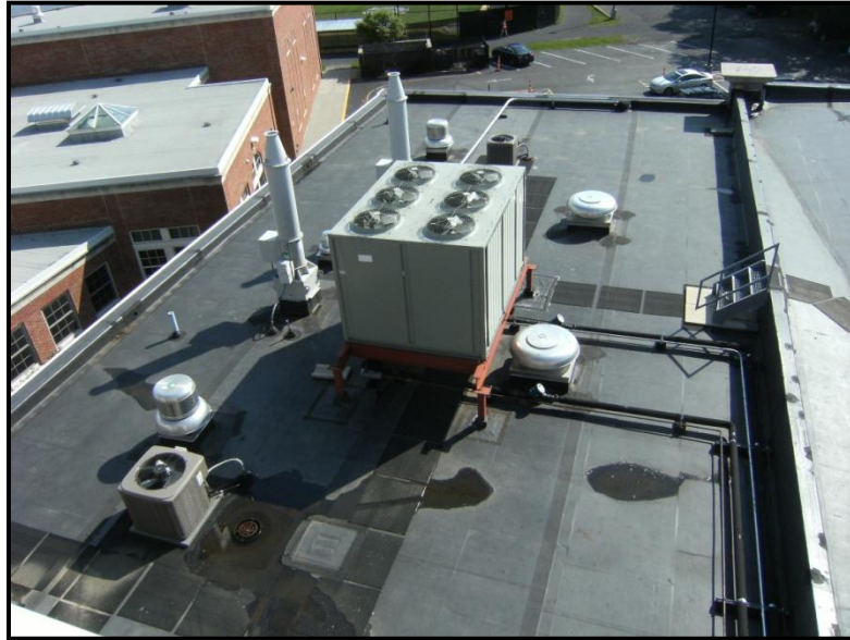
Figure 38: Auditorium Condensing Unit
