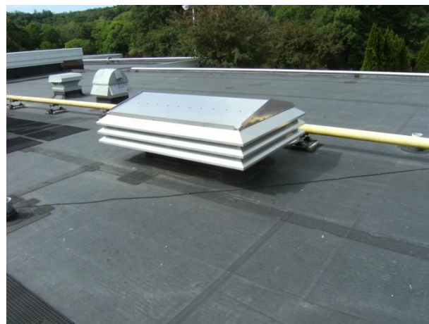
Figure 4: Typical 1954 Wing – Gravity Roof Outlet
