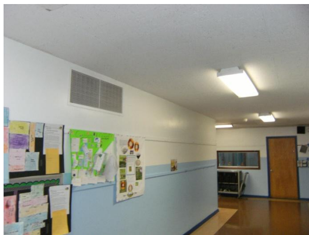
Figure 14: 1961 Wing Corridor Exhaust Transfer Grille
