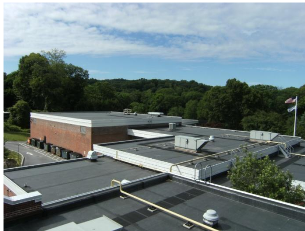
Figure 6: Two Library Roof Top Units
