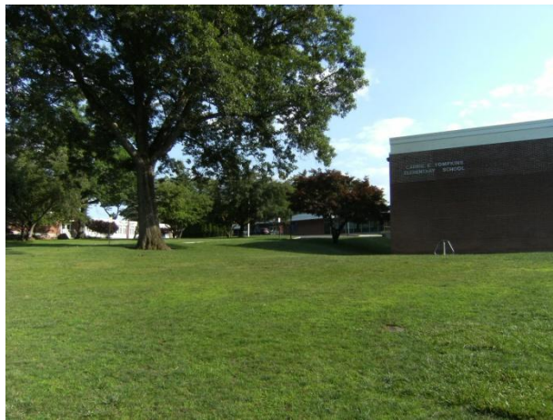
Figure 1: CET Elementary School
