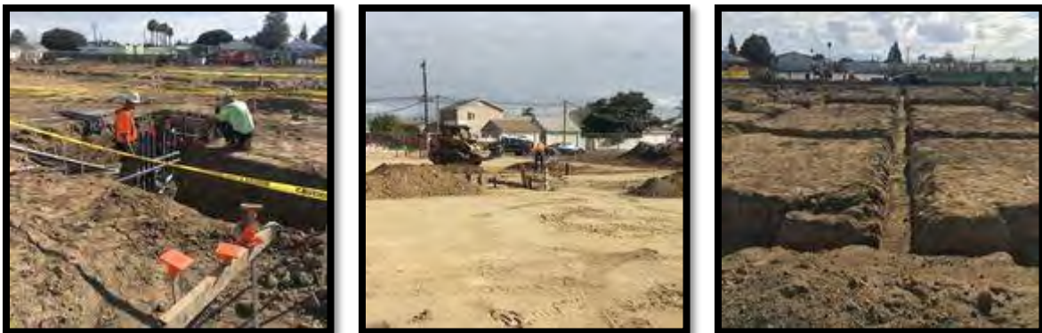
Reconstruction of McKinna School – November 2018
