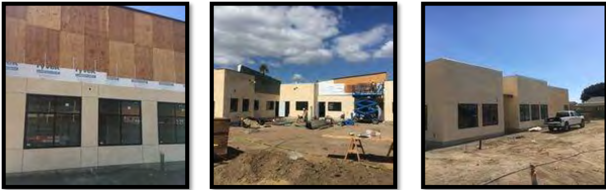
Lemonwood Elementary School Construction Progress – November 2018
