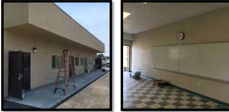
Brekke Kindergarten/Flex Classroom Building Construction Progress – November 2018
