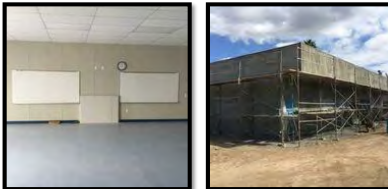
Ritchen Kindergarten/Flex Classroom Building Construction Progress – November 2018
