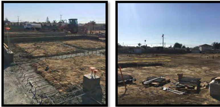
Ramona Kindergarten/Flex Classroom Building Construction Progress – November 2018
