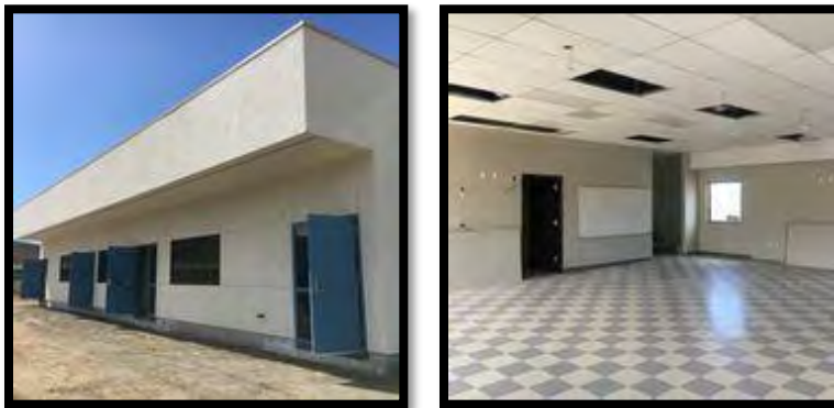
McAuliffe Kindergarten/Flex Classroom Building Construction Progress – November 2018
