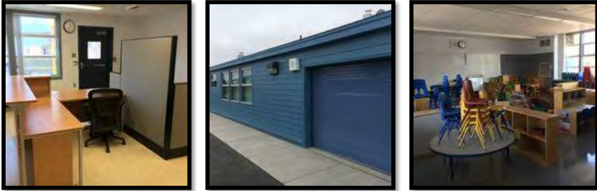
Harrington Kindergarten Annex Construction Progress – November 2018
