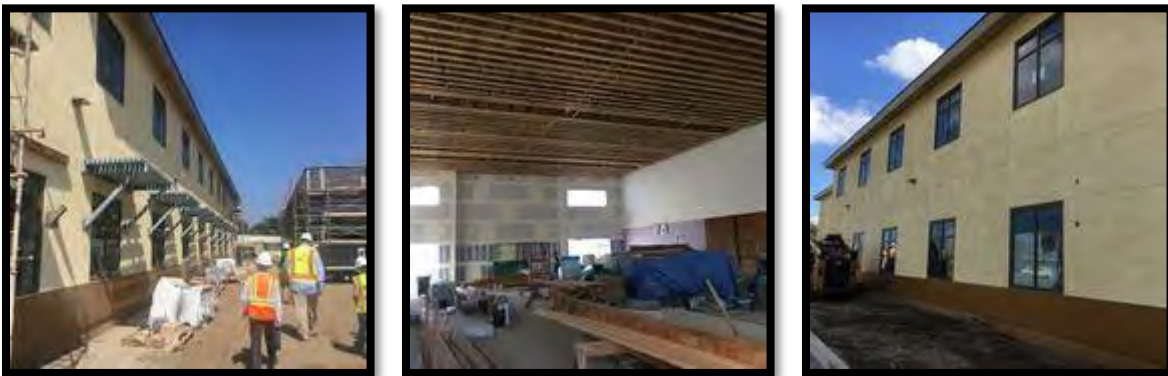
New Elm School Construction Progress – November 2018
