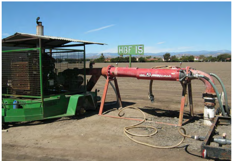
Photograph 6: View of pumping station adjacent to the south of the site.
