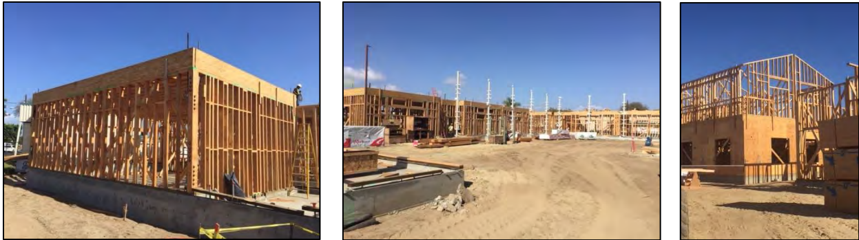
New Elm School Construction Progress – November 2017
