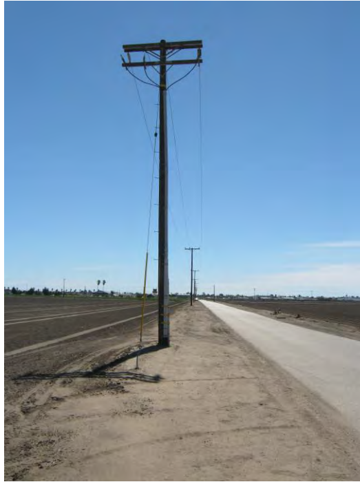
Photograph 3: View of power lines on the western portion of the site.
