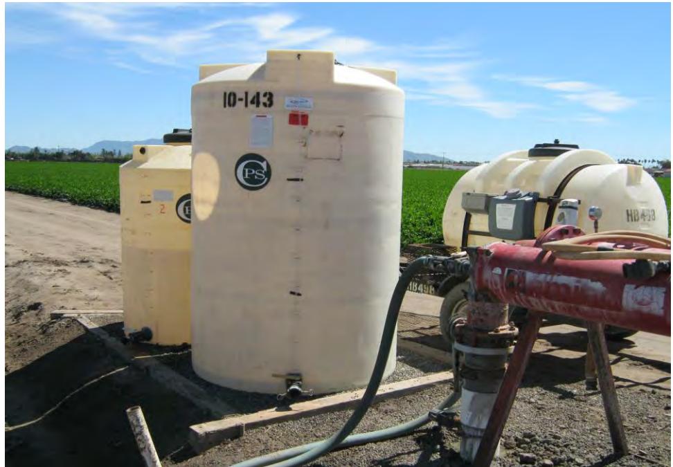
Photograph 7: View of 1,000-gallon empty AST and two 500-gallon ASTs (one mobile unit) labeled as containing phosphoric acid, potassium chloride, and nitrogen.
