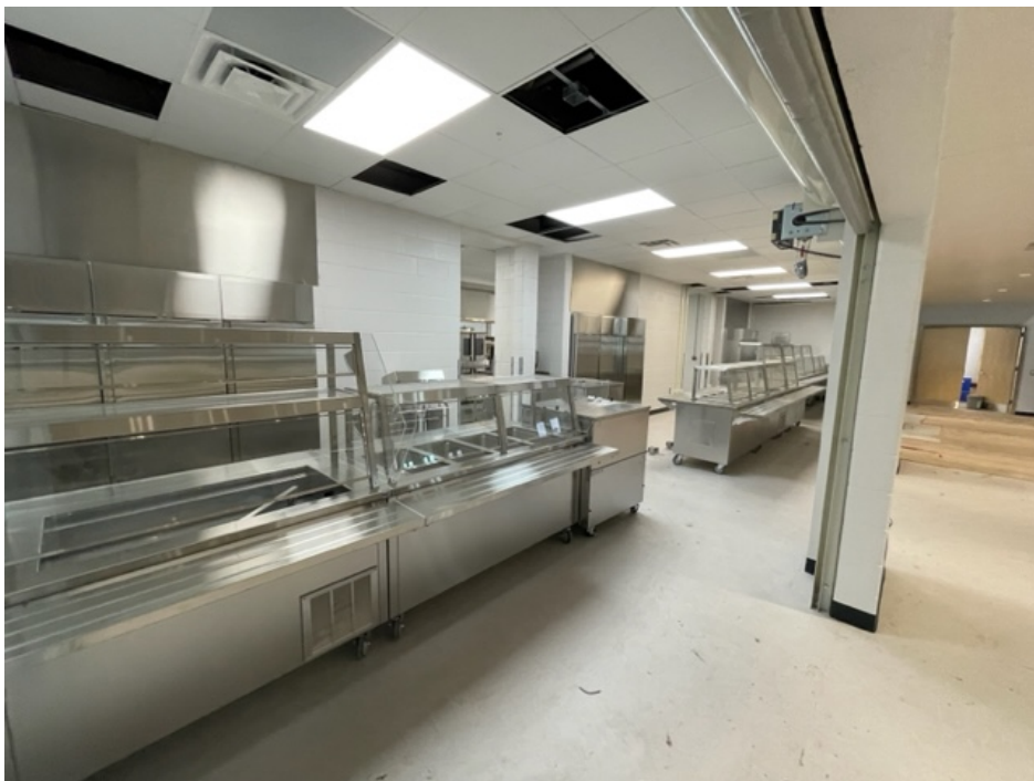
Kitchen - plumbing hook-ups this week.
