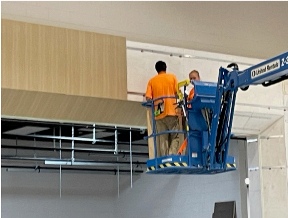
Trim being installed over Stage area in Caffeterium
