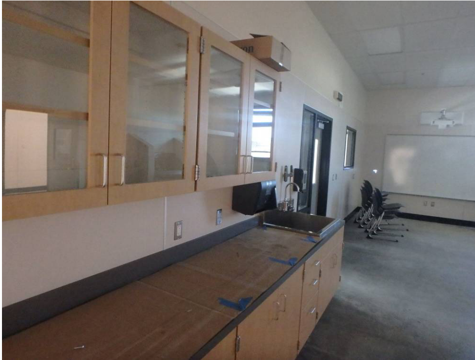
Lab – looking south at the east wall
