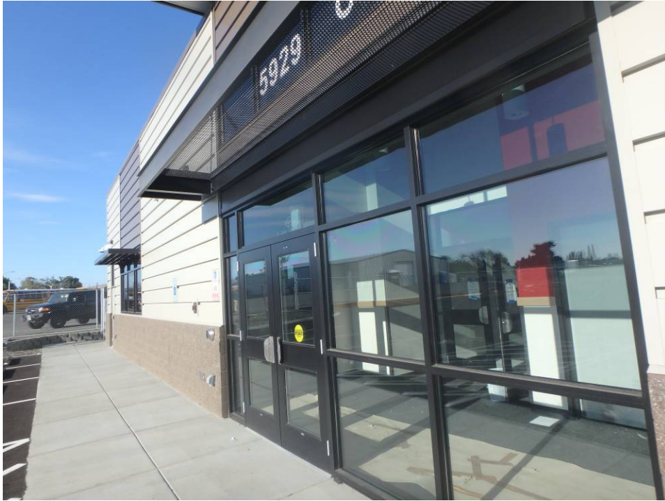
Main entry doors and sidelites interior view
