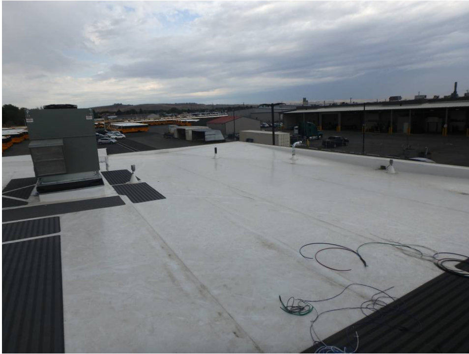
Looking at the southwest corner of the roof (7/10/23)
