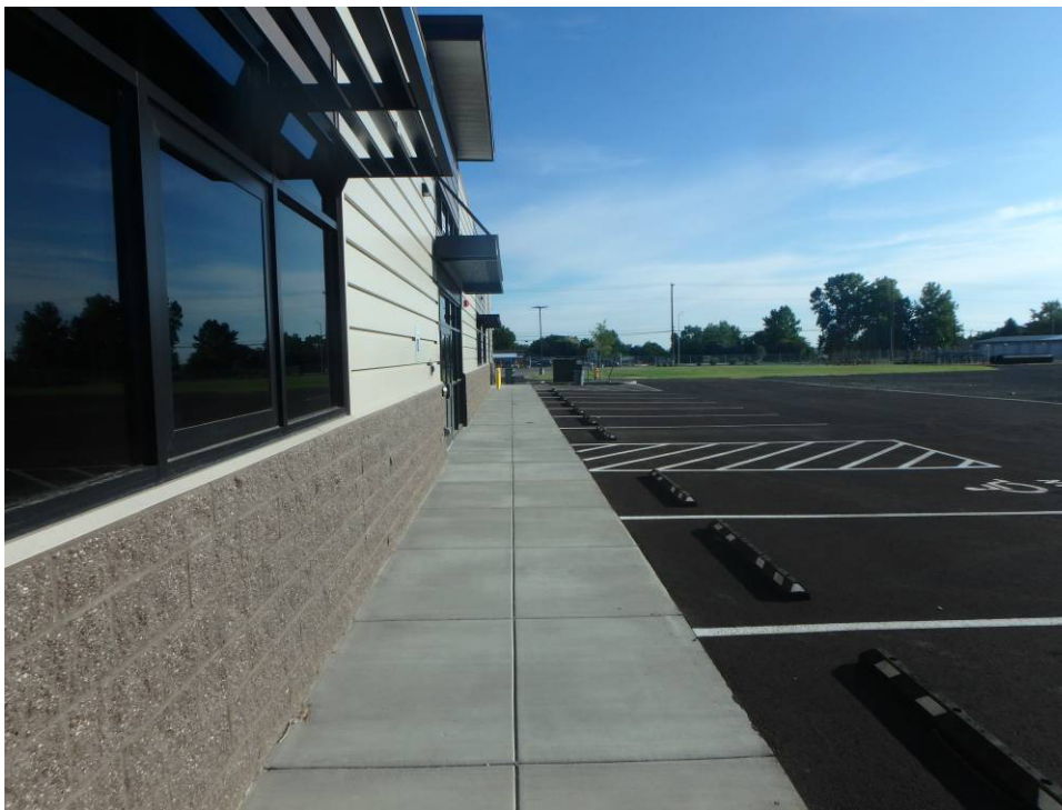
Looking north along the front of the building
