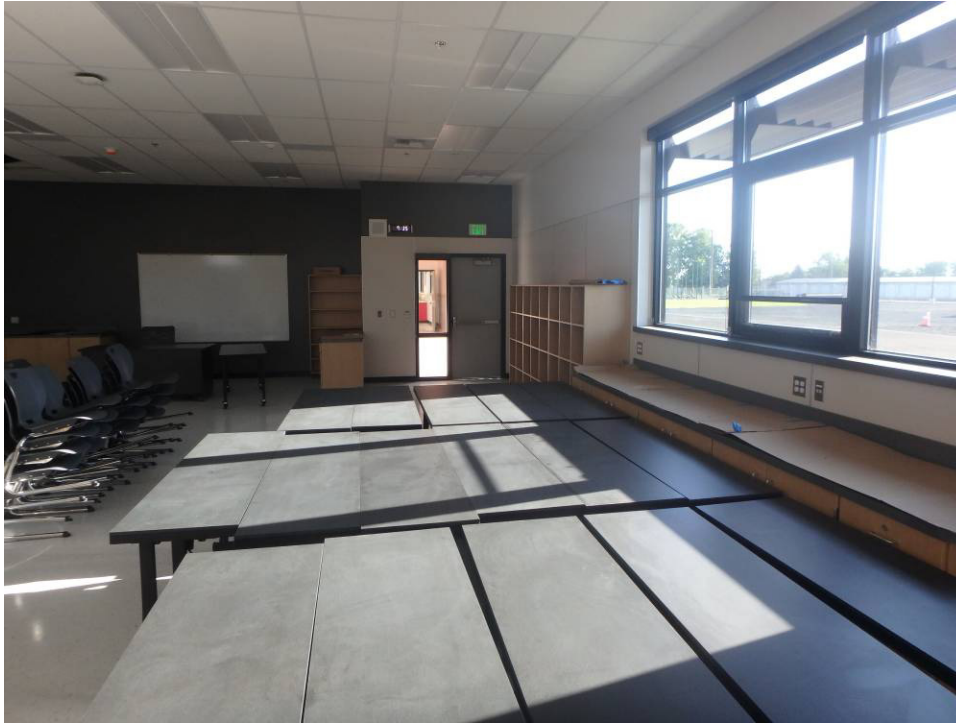
Looking north at the casework at the east wall of the south classroom
