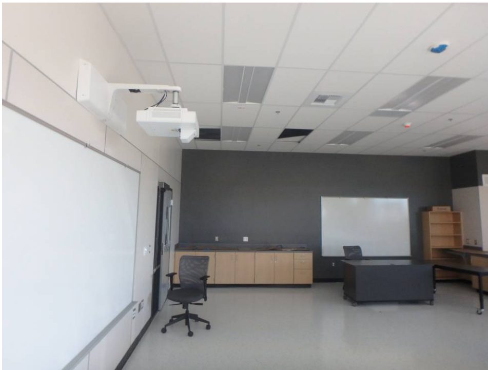
Looking at the casework in the northwest corner of the south classroom
