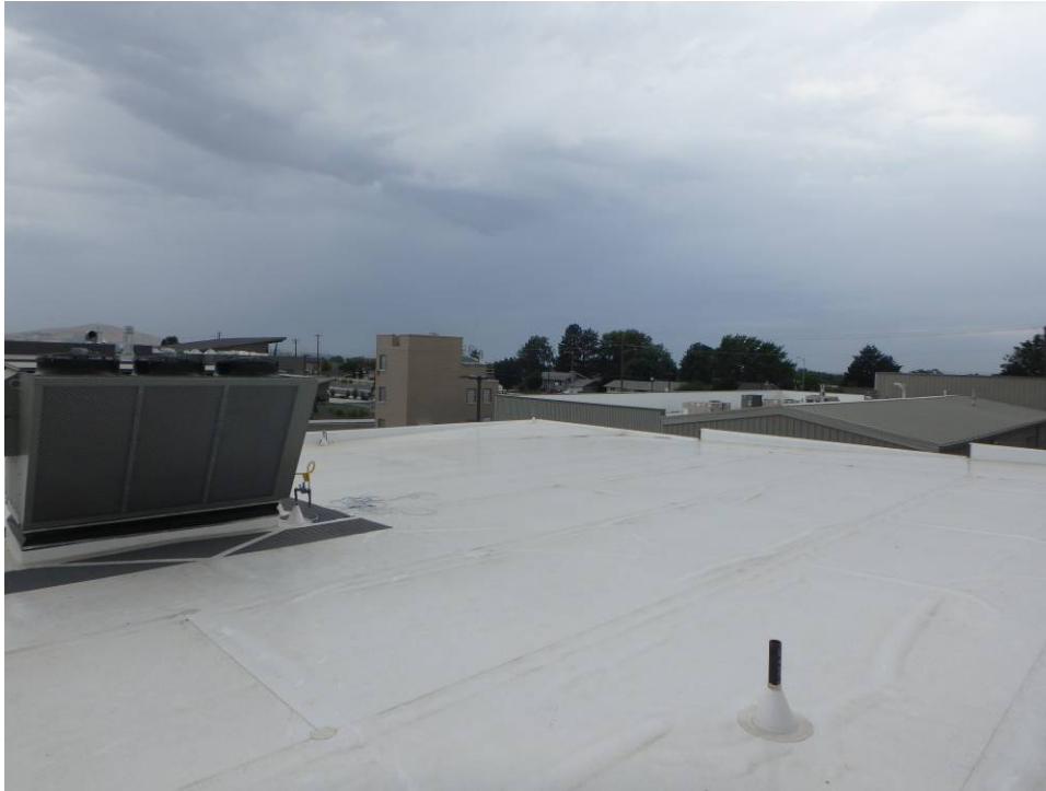
Looking at the northwest corner of the roof (7/10/23)
