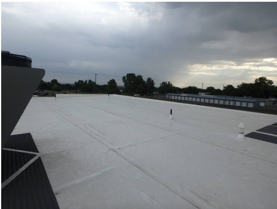
Looking at the northeast corner of the roof (7/10/23)
