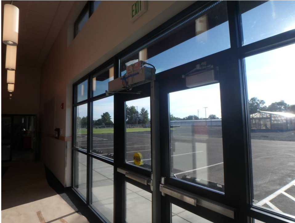
Main entry doors
