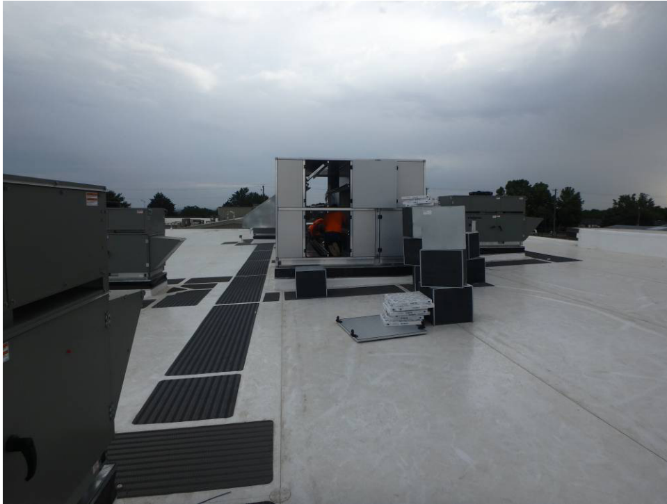
Installing ERV filter and exchanger boxes from south (7/10/23)
