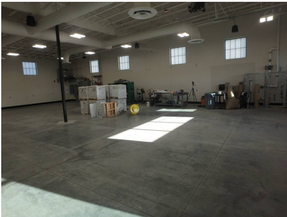
Looking northwest into the shops northwest corner
