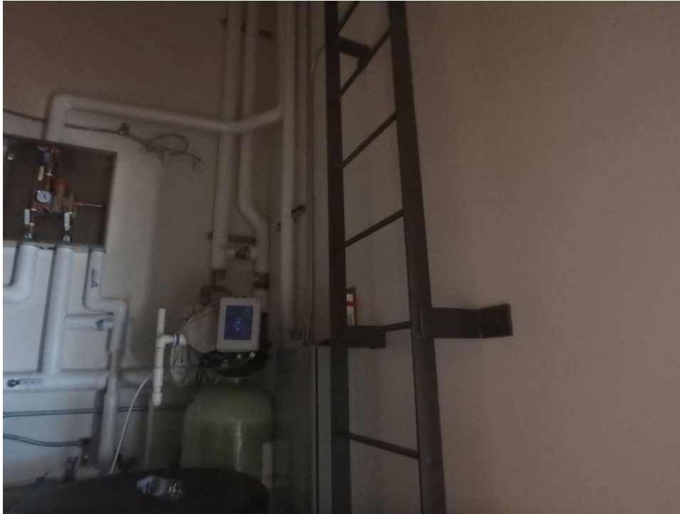
Mechanical room – Piping revision area
