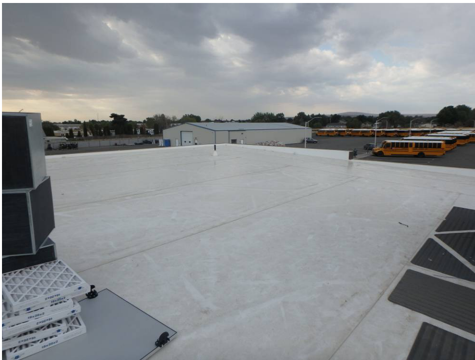
Looking at the southeast corner of the roof (7/10/23)
