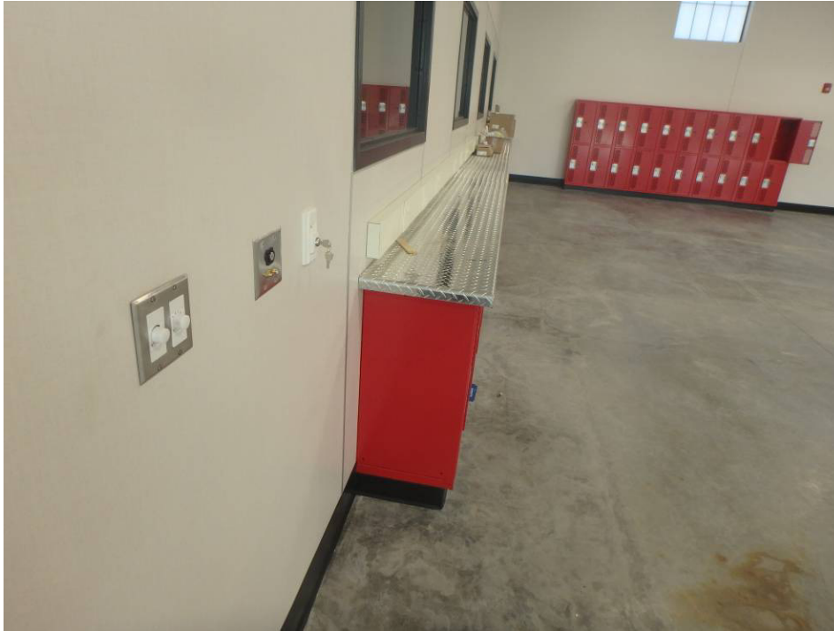
Looking west at the shop's south wall
