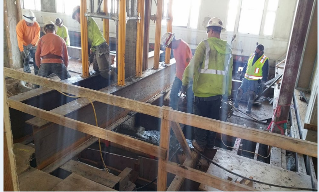
New foundation under existing columns
