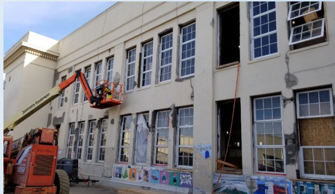
Repair exterior walls and windows
