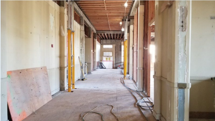
Repair of upper flooring/ceiling
