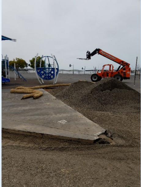
New ADA* Ramp
