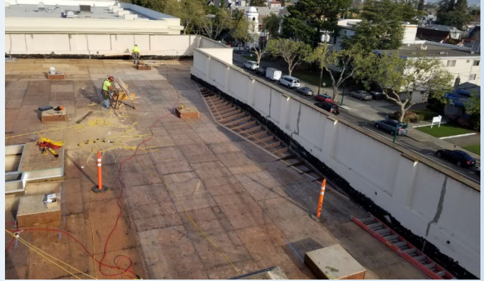
New structural roof at Central Building
