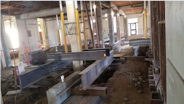
New footings/foundation to support the second floor
