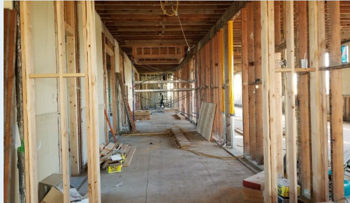
Framing of classroom building
