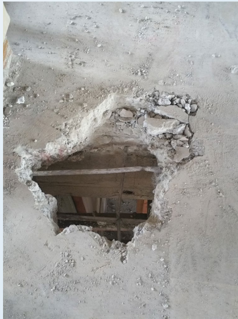
Removal of floor & concrete testing per DSA
