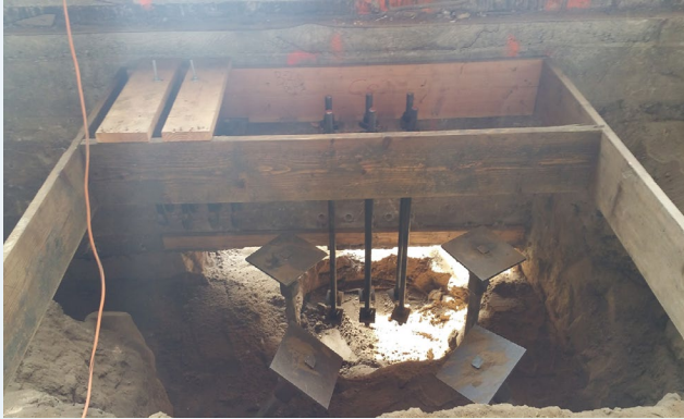
New foundation with anchor rods and helical piles
