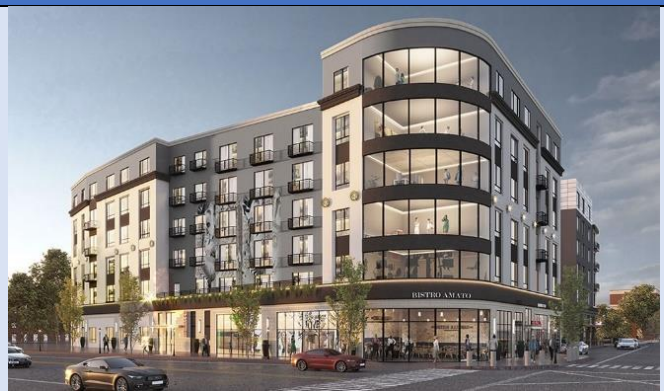
The Highrailer 114 Units (3% LMI)
