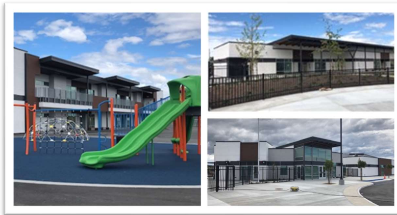
Reconstructed McKinna Elementary School
