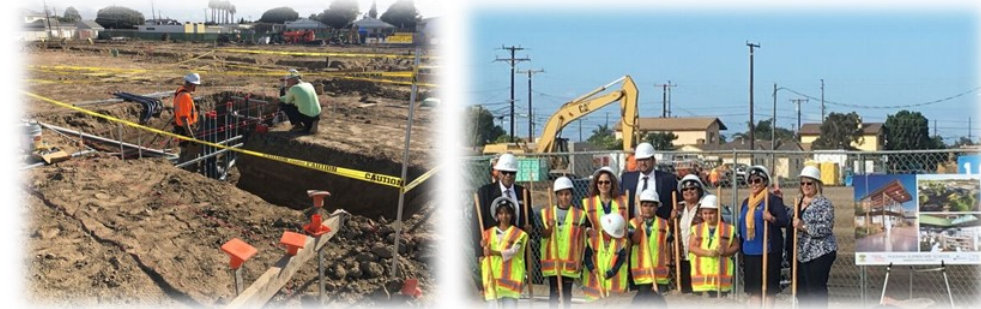
McKinna Elementary School Construction Progress (Left) and Groundbreaking (Right)
