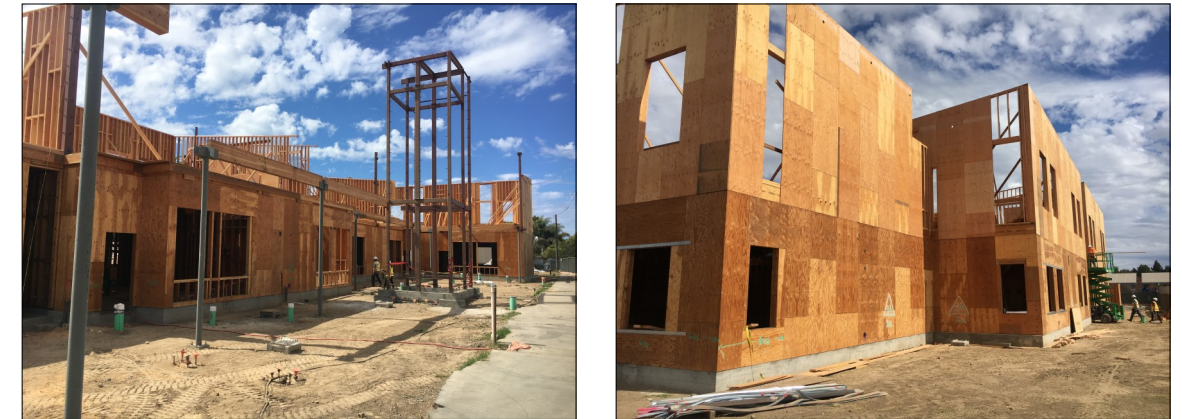
New Marshall Classroom Building Construction Progress - October 2018
