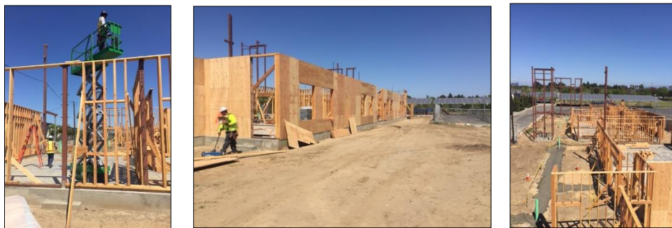
Marshall New Classroom Building Construction Progress – May 2018
