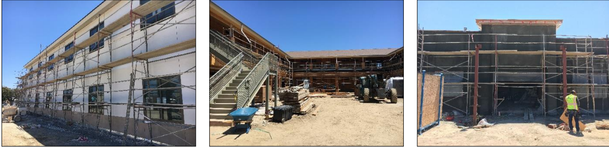
New Elm School Construction Progress – May 2018
