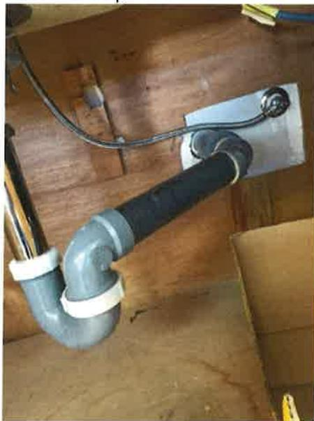
Kiwitt General Building will replace the incorrect waste line that was installed under the sink and replace with the cpvc pipe that was approved. our supplier issued us the wrong pipe and will reimburse us for the pipe that they gave us.
