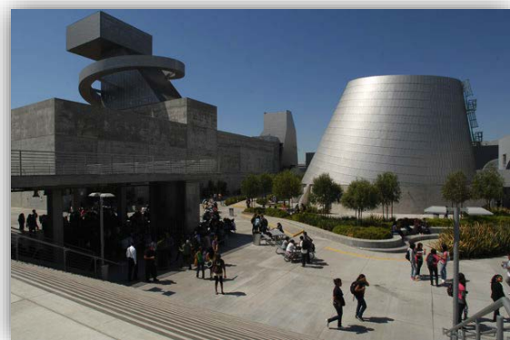
The completed LAUSD New High School #9, where the efforts of the Parsons PSA management team helped keep work going during the crane operators strike in the Summer of 2007.
