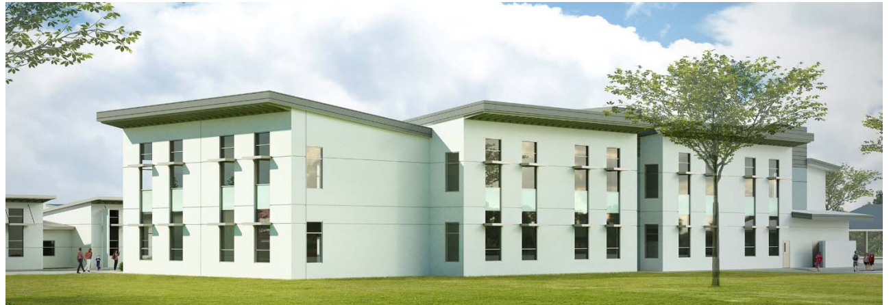
Marshall New Classroom Building February 3, 2016
