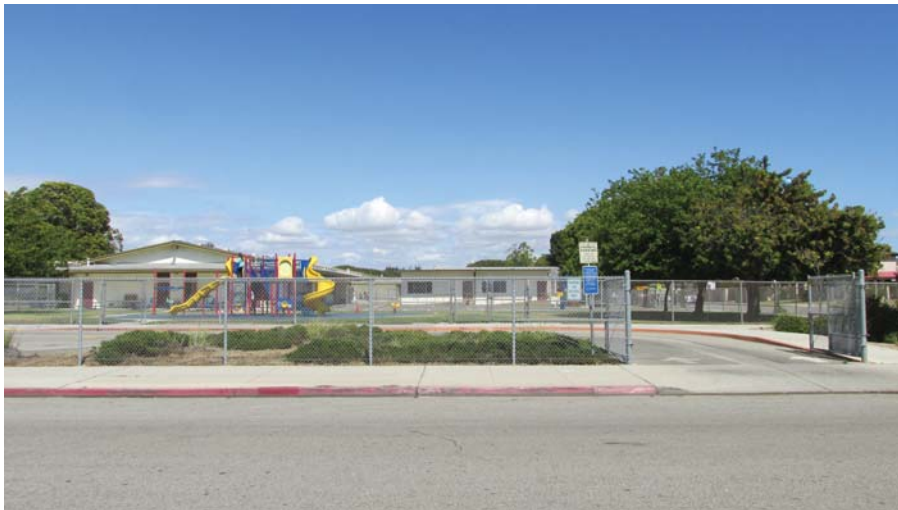
Photo 2: Existing Front of School and Loading Zone
