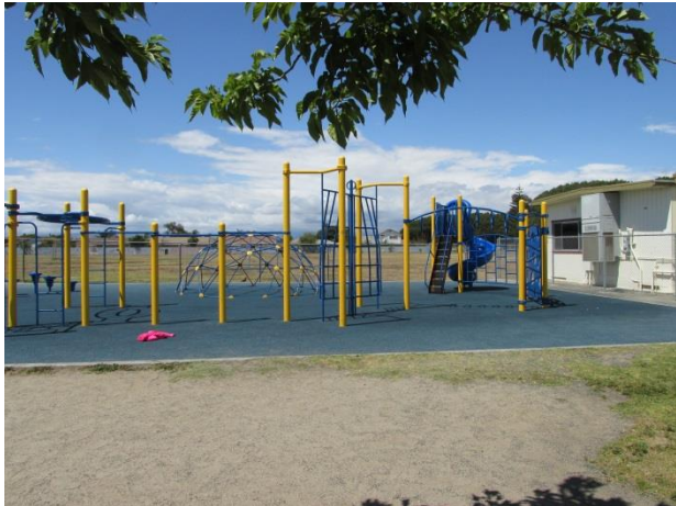
Photograph 3. View of playground.
