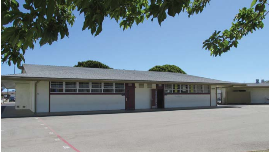
Photo 1: Existing School Building
