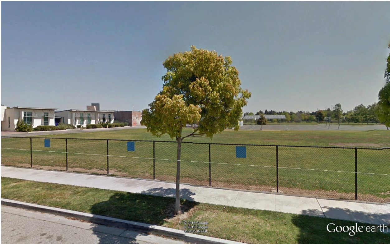
Figure 3-1. Image of Existing School Buildings (Google Earth 2015)
