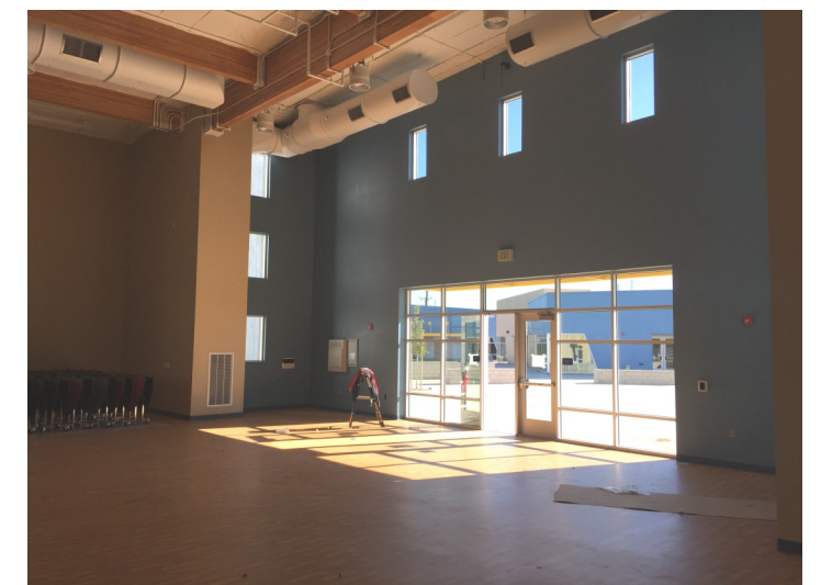
New Norma Harrington Multipurpose Building
