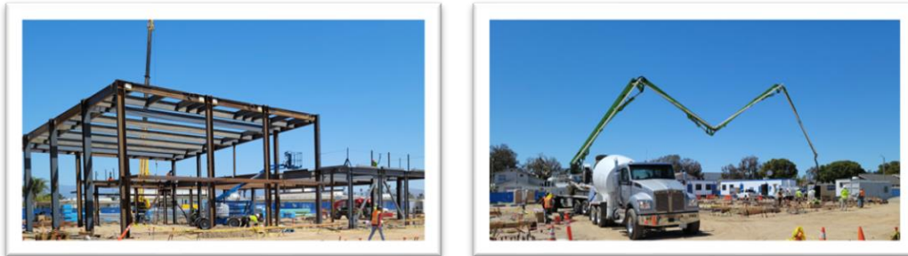
Rose Avenue Elementary School Construction Progress
