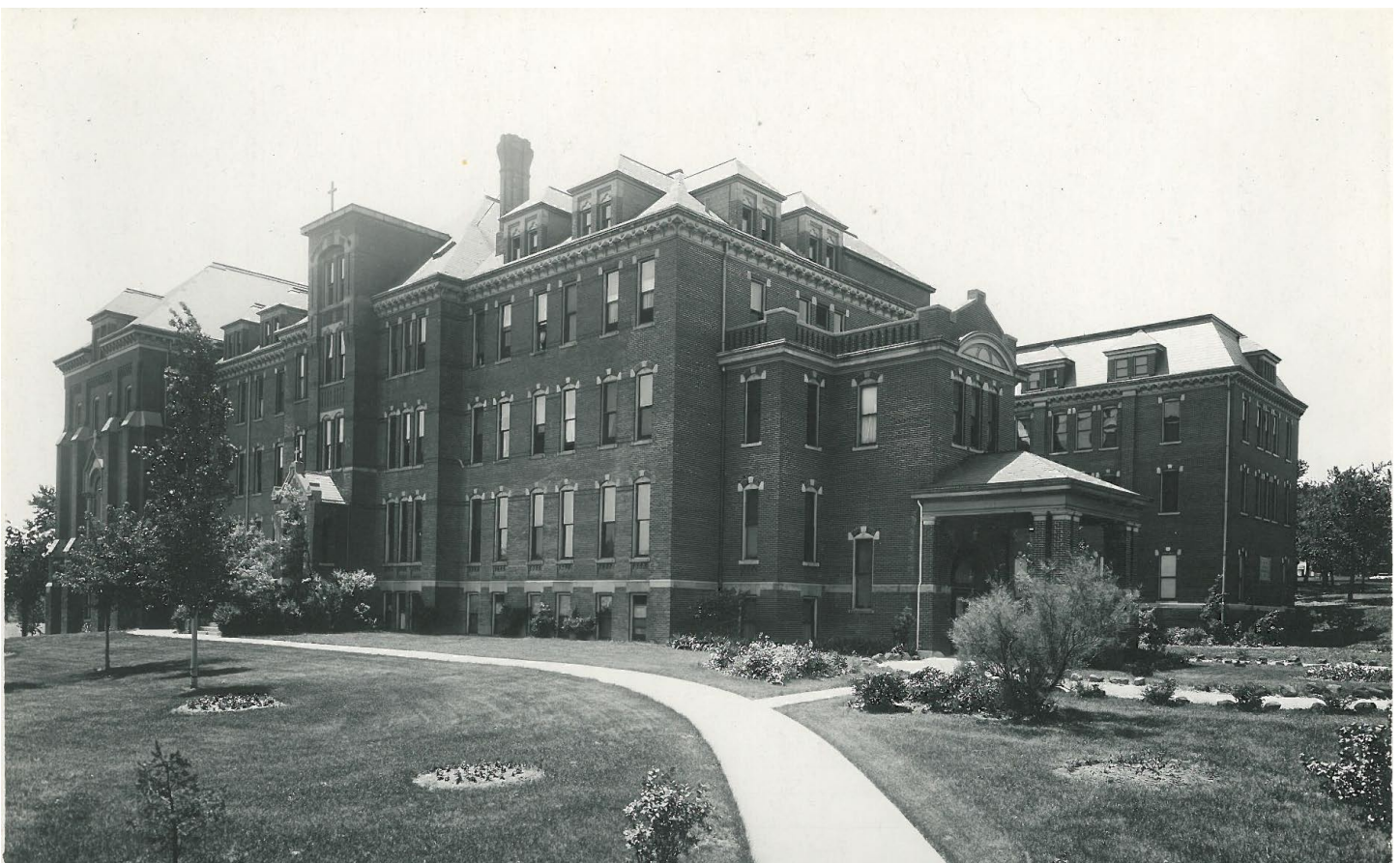
Photo G: This photo shows the 1920 building (far right) and how the North Face of Duchesne and circle drive was changed to its present look. Notice the hip roof over the 3 story chapel. The 4 th floor was added in 1930.
