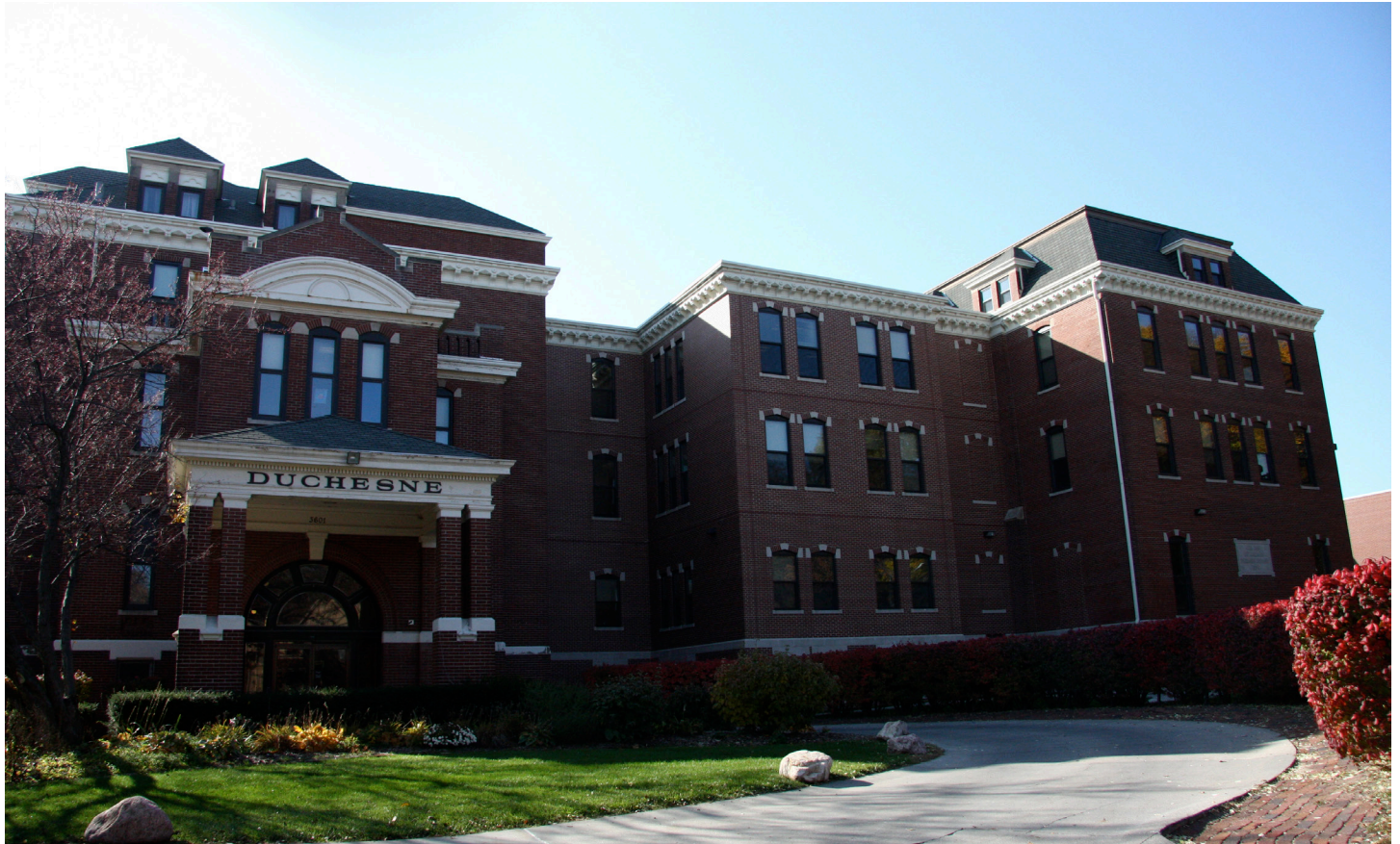
A exterior view of the completed "connector" building constructed in 2003.
