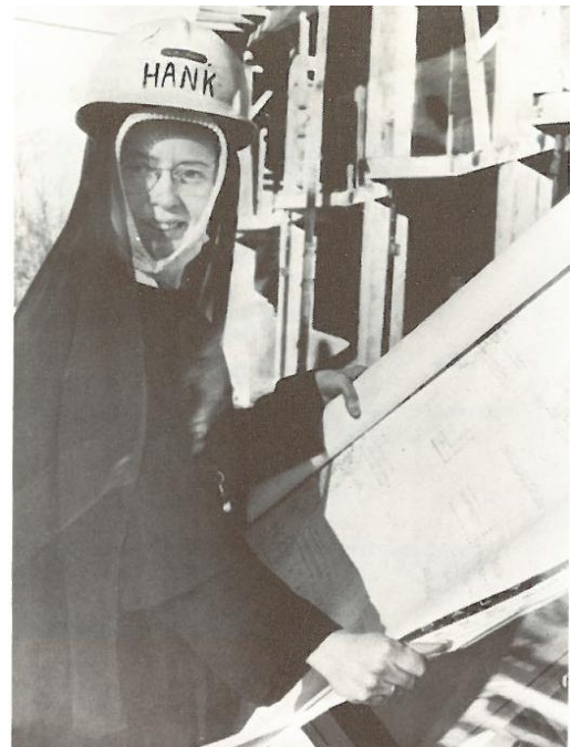
Photo M: Mother Catherine Henry inspecting the construction of Matthews Hall.
