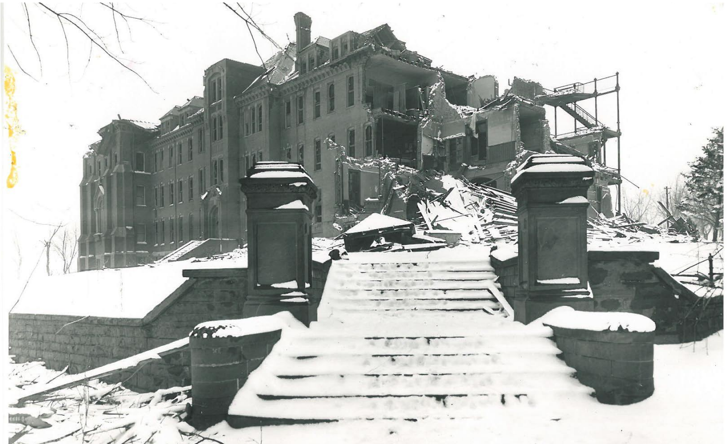
Photo F: The Easter Tornado of 1913 destroyed the north wing. In this picture you can also see the damage to the roof above the chapel.
