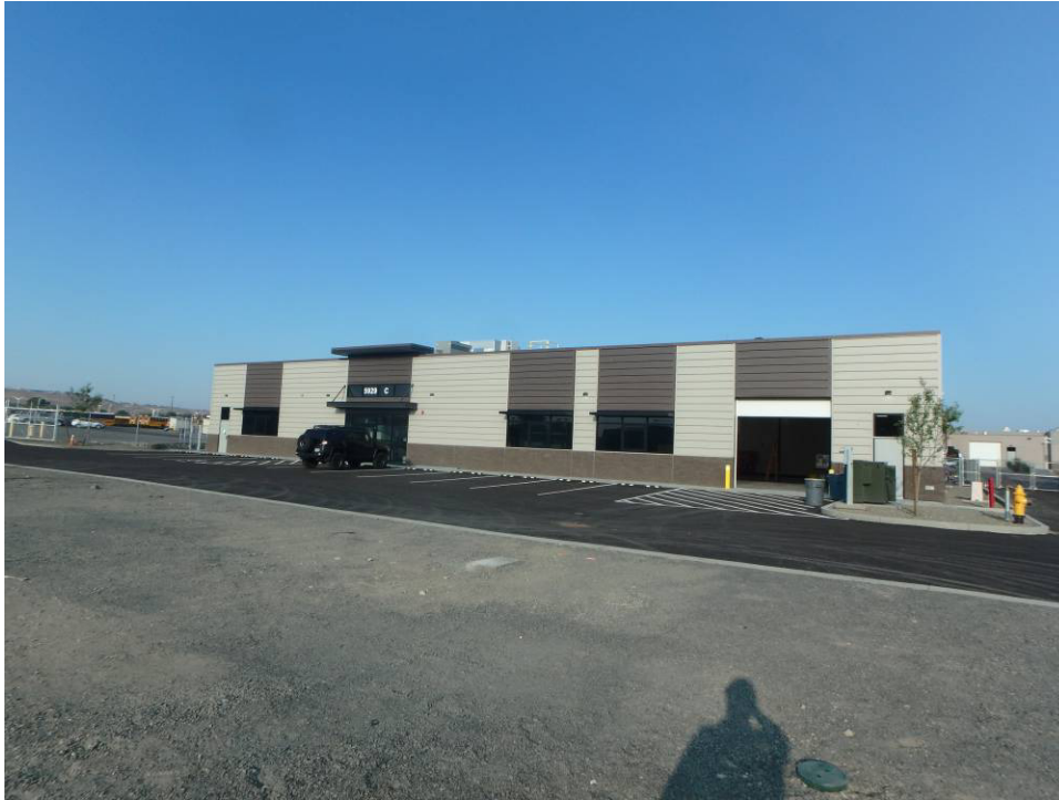
Looking west at the northeast corner of the building
