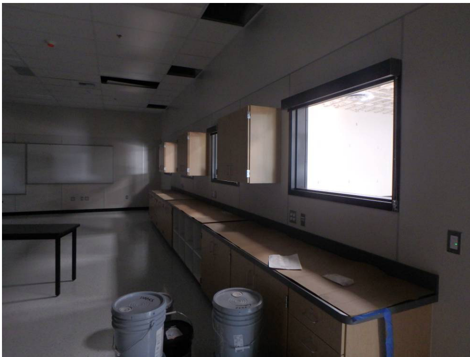
Looking west at the north wall of the north classroom
