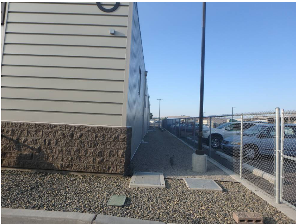
Looking south along the west edge of the building (6/27)
