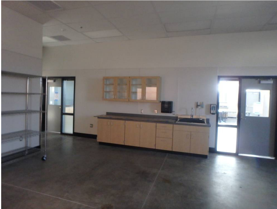
Lab – eyewash station and east wall
