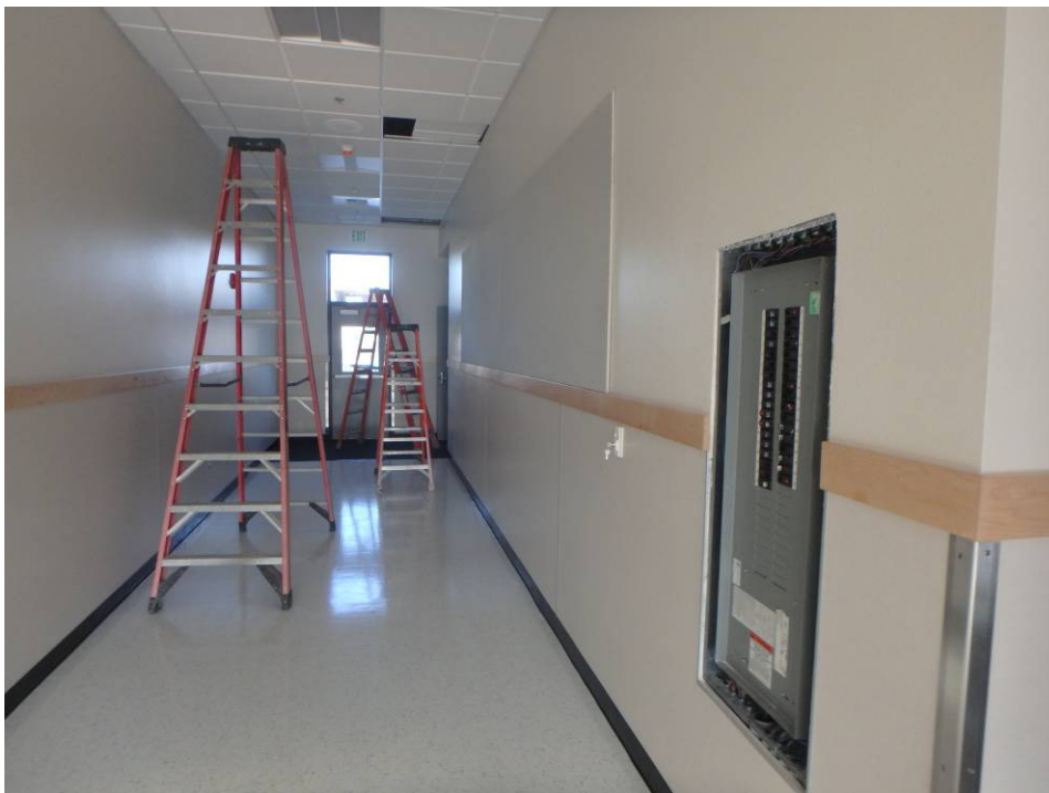
Looking west at the main east-west corridor
