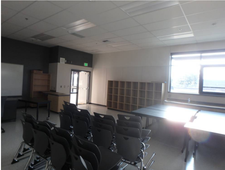
Looking at the casework at the east wall of the south classroom - north
