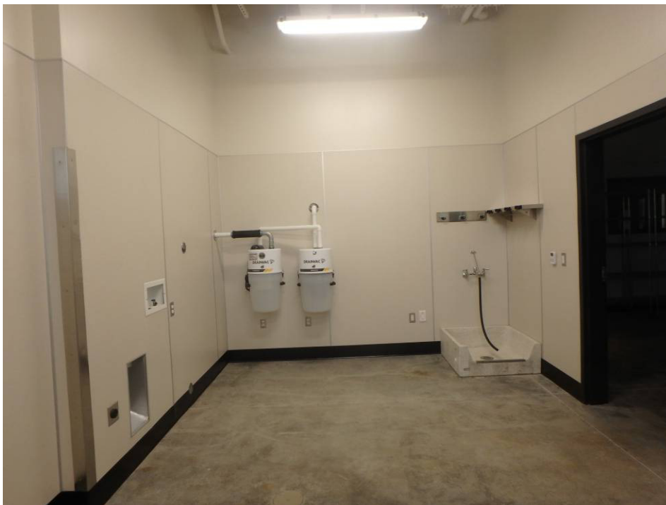
Kennel Room vacuum and janitor sink on the north wall
