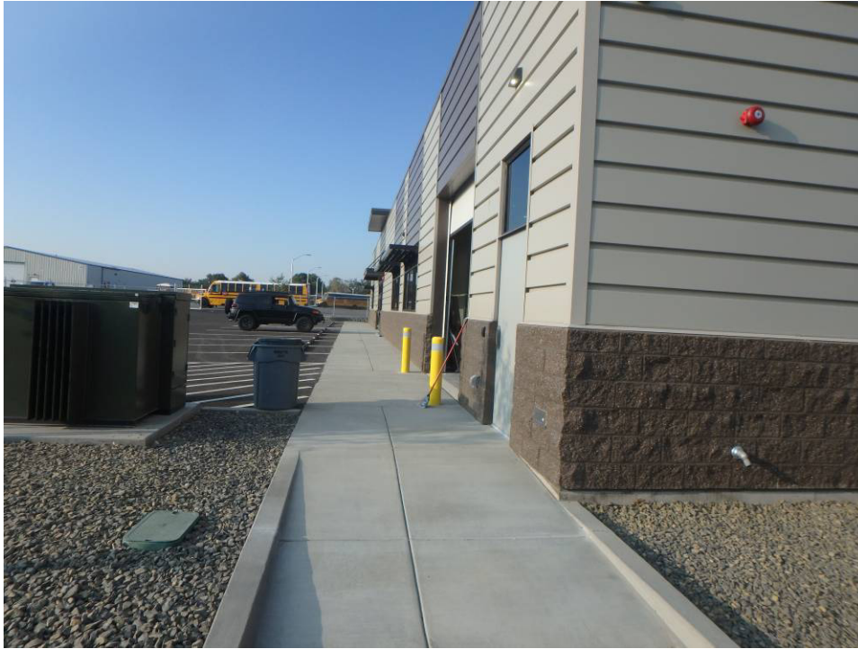
Looking south along the east edge of the building
