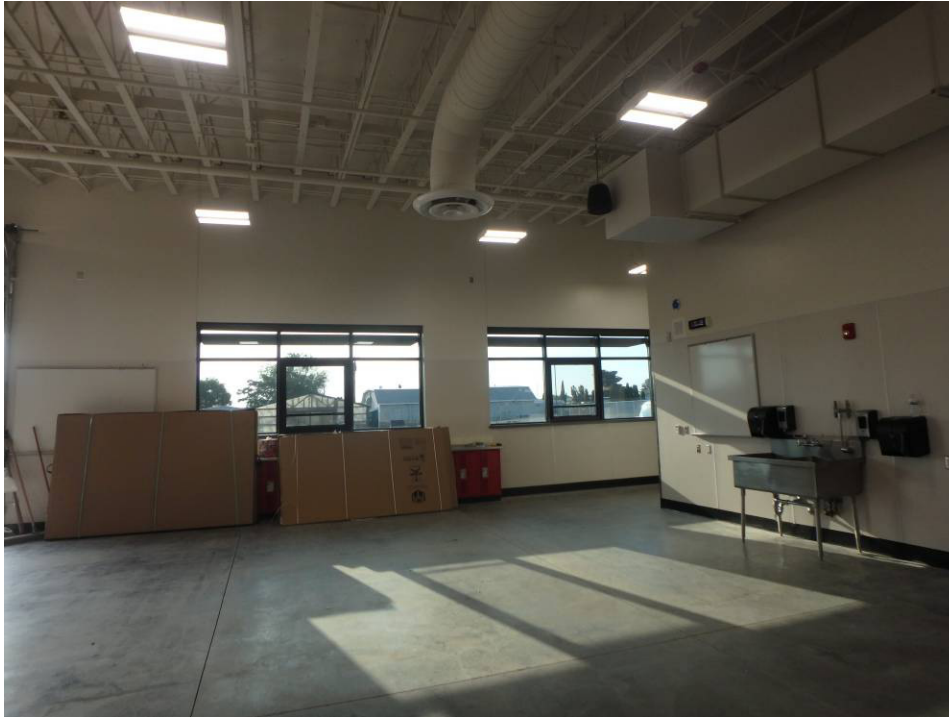
Looking east at the shop's south wall
