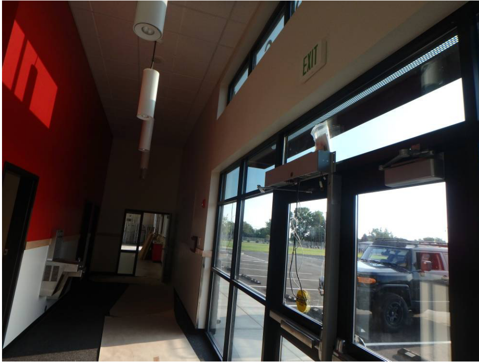
Main entry doors and sidelites interior view
