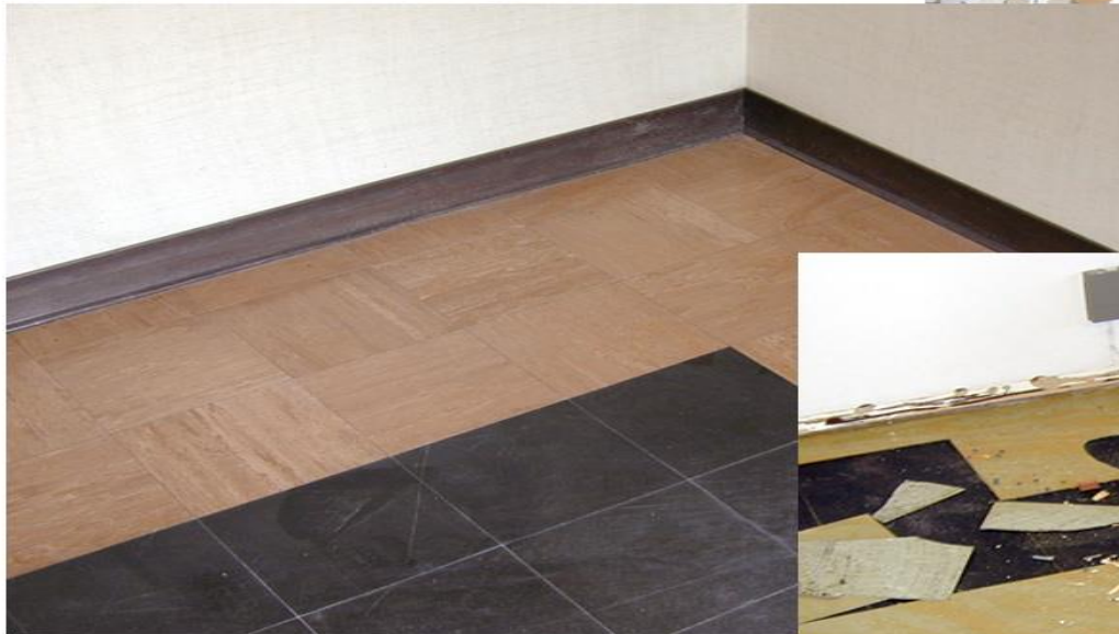
9" VINYL ASBESTOS TILE (LEFT) & BLACK ASBESTOS MASTIC (BELOW) EXPOSED DURING CARPET REMOVAL
