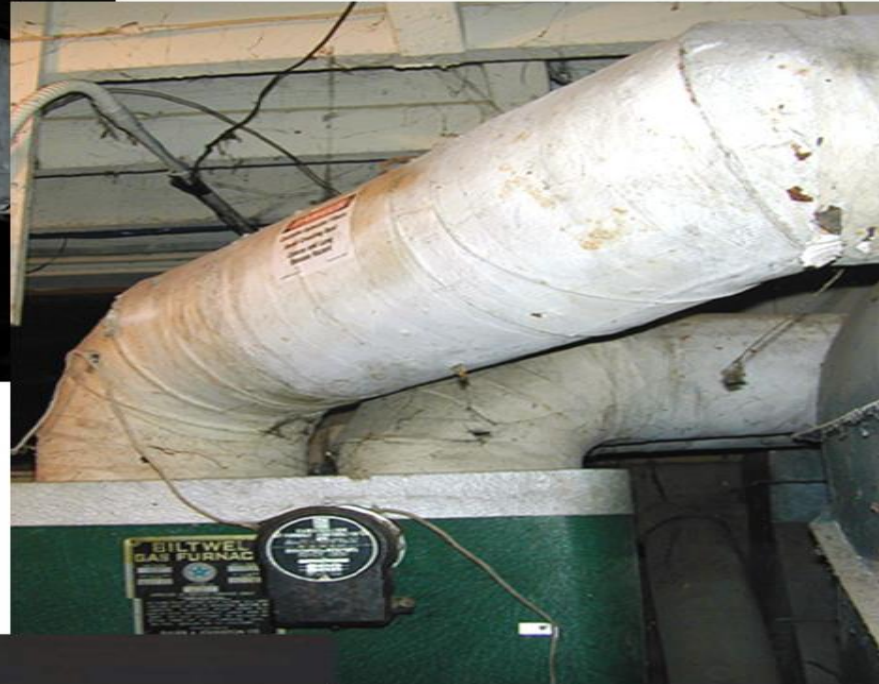
CORRUGATED (ABOVE) AND FLAT (RIGHT) ASBESTOS PAPER ON FURNACE DUCTS
