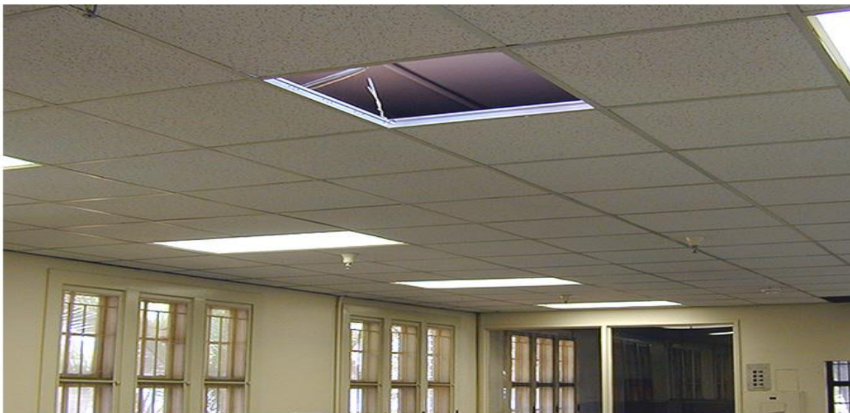
LAY-IN ACOUSTIC CEILING TILE
