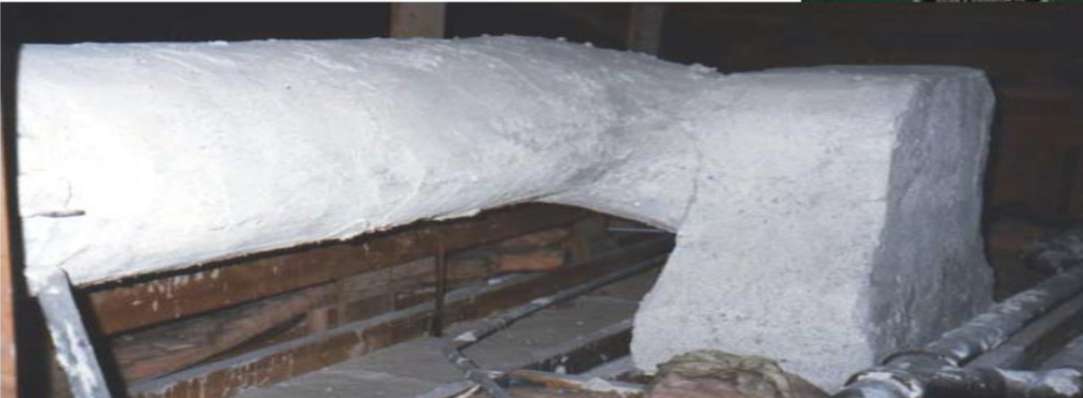
TROWELED-ON INSULATION ON KITCHEN HOOD EXHAUST DUCT
