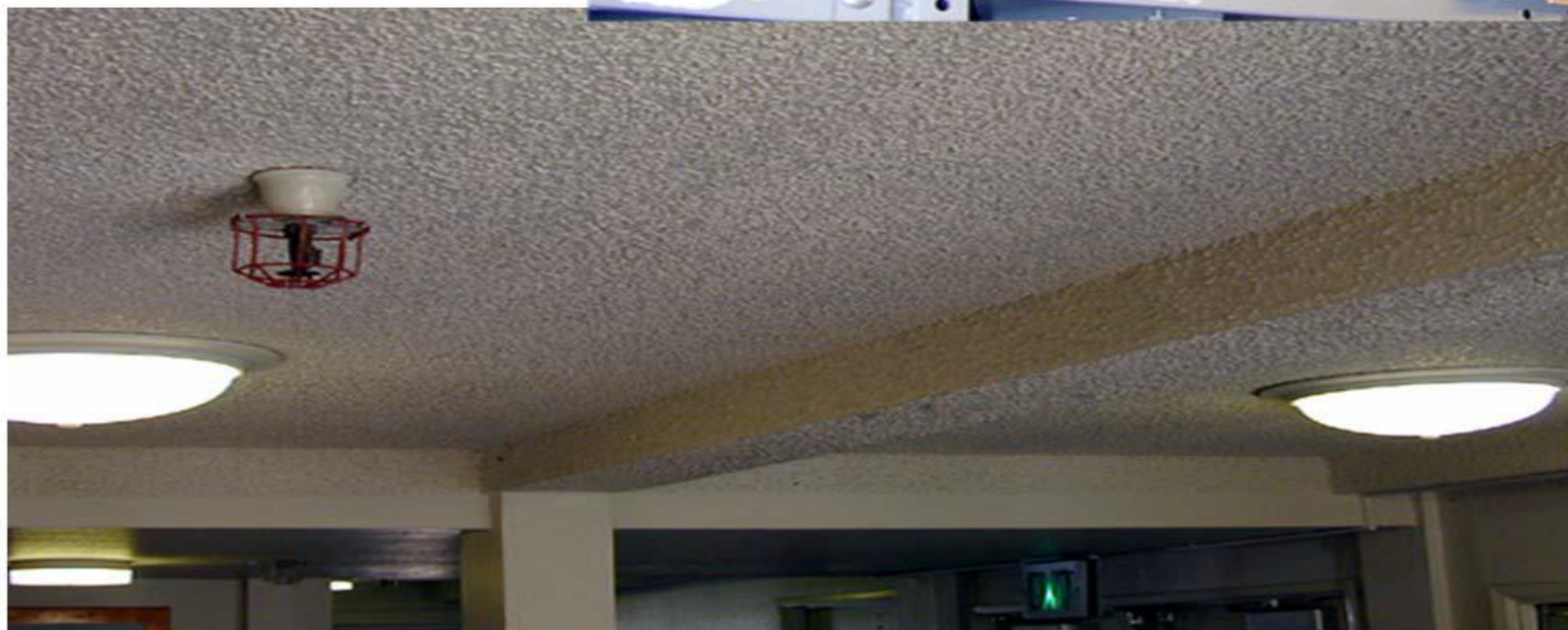
SPRAY-APPLIED ACOUSTIC CEILING PLASTER
