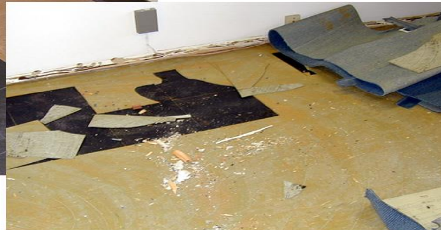
9" VINYL ASBESTOS TILE (LEFT) & BLACK ASBESTOS MASTIC (BELOW) EXPOSED DURING CARPET REMOVAL
