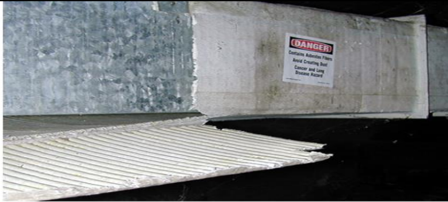
CORRUGATED (ABOVE) AND FLAT (RIGHT) ASBESTOS PAPER ON FURNACE DUCTS
