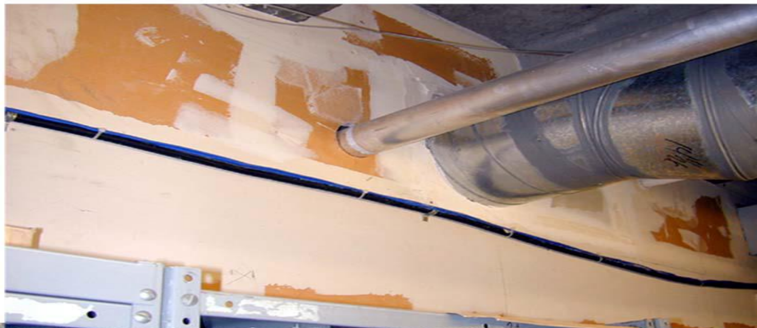
JOINT COMPOUND OVER SHEETROCK WALLBOARD
