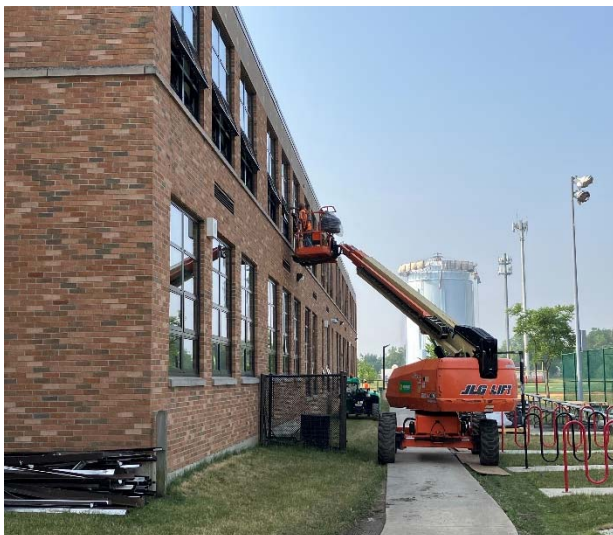
Left: New window installation is progressing along the second floor.
