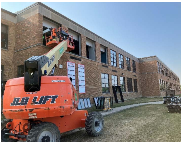
Left: New windows being installed on the second floor.
