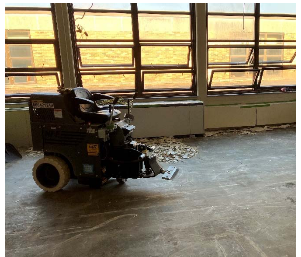
Right: A riding scraper is used to clear large areas of tile flooring in a second floor classroom.
