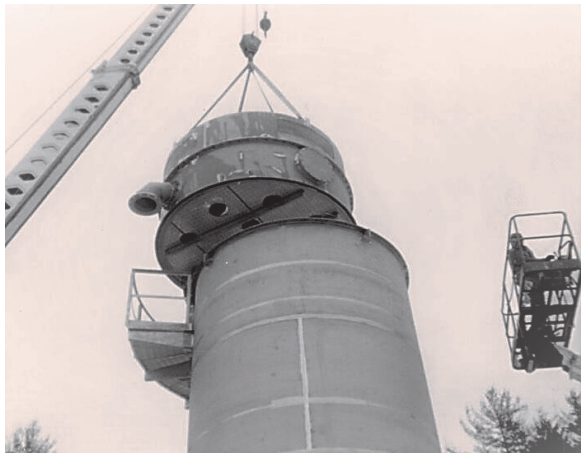
The Hendrick Street Water Treatment Facility Assembling the Aeration Tower 1996
