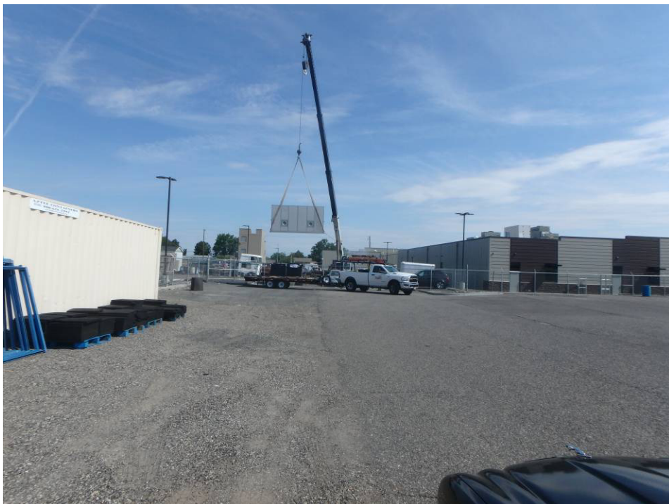
Lifting second panel (6/27)
