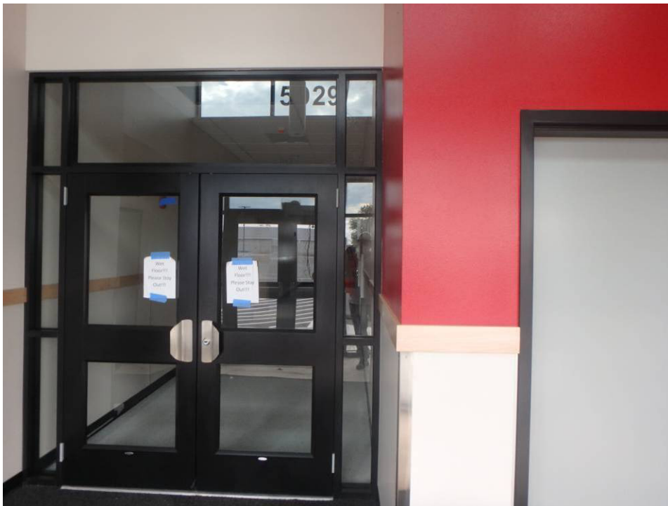
Vestibule doors to e-w corridor
