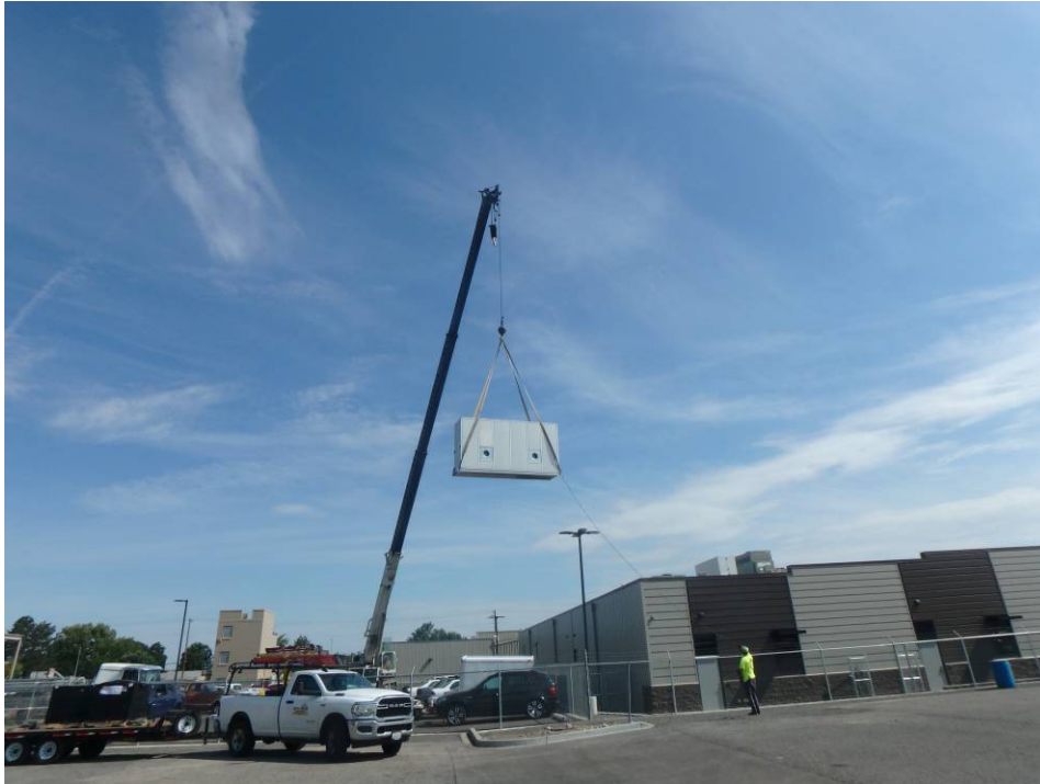
Lifting second panel (6/27)
