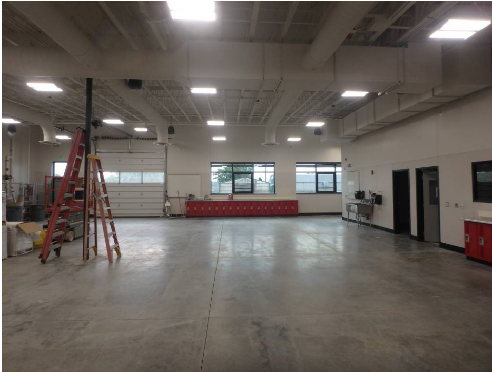
Looking east at the shop's south wall
