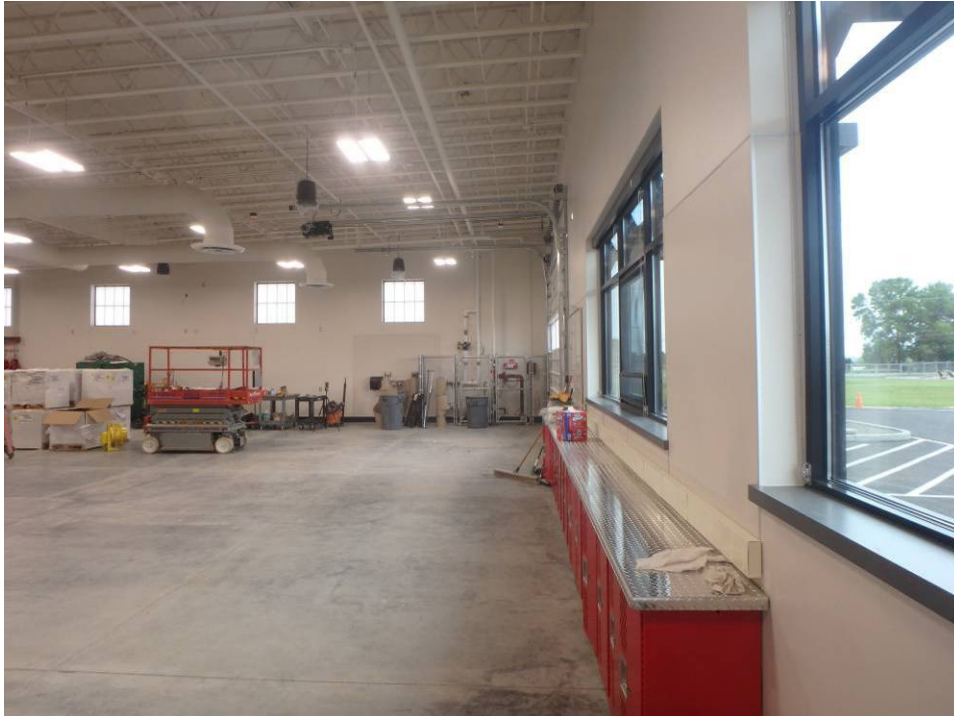
Looking north along the shop's east wall and lockers with diamond plate top
