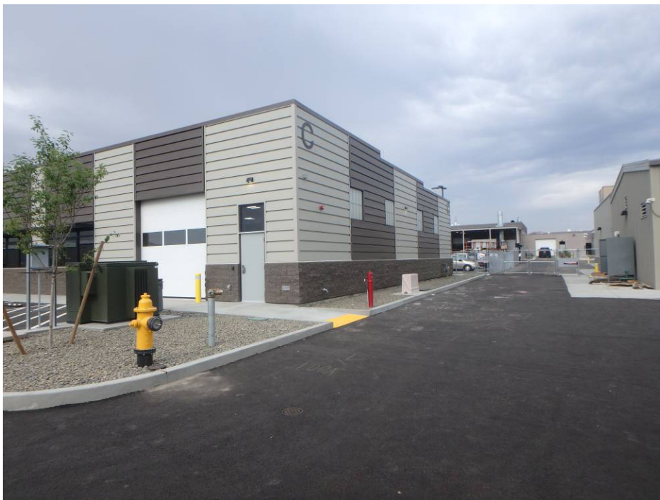
Looking at the northeast corner of the building
