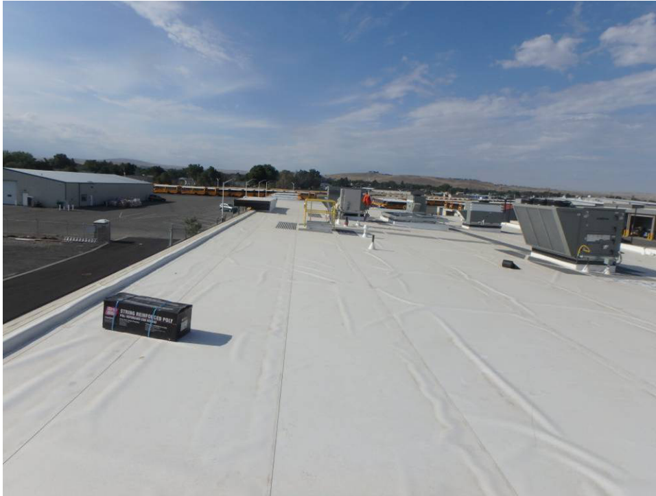
Looking south along the east edge of the building (6/27)
