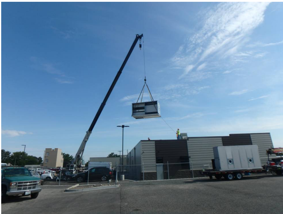
Lift DOAS to building (6/27)
