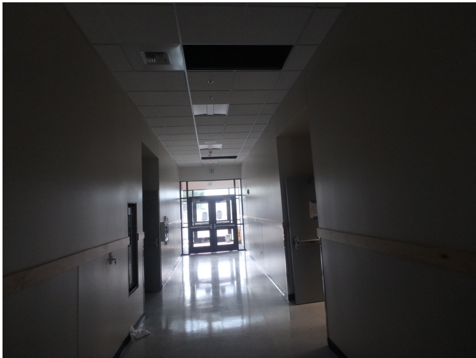
Looking east at the main east-west corridor
