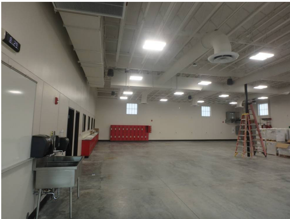
Looking west along the south wall of the shop
