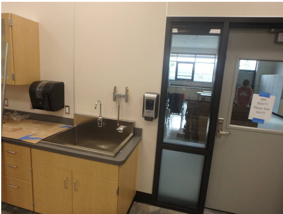
Lab – eyewash station and east wall
