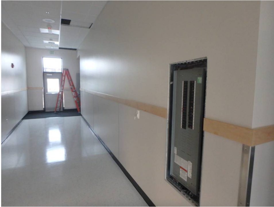
Looking west at the main east-west corridor
