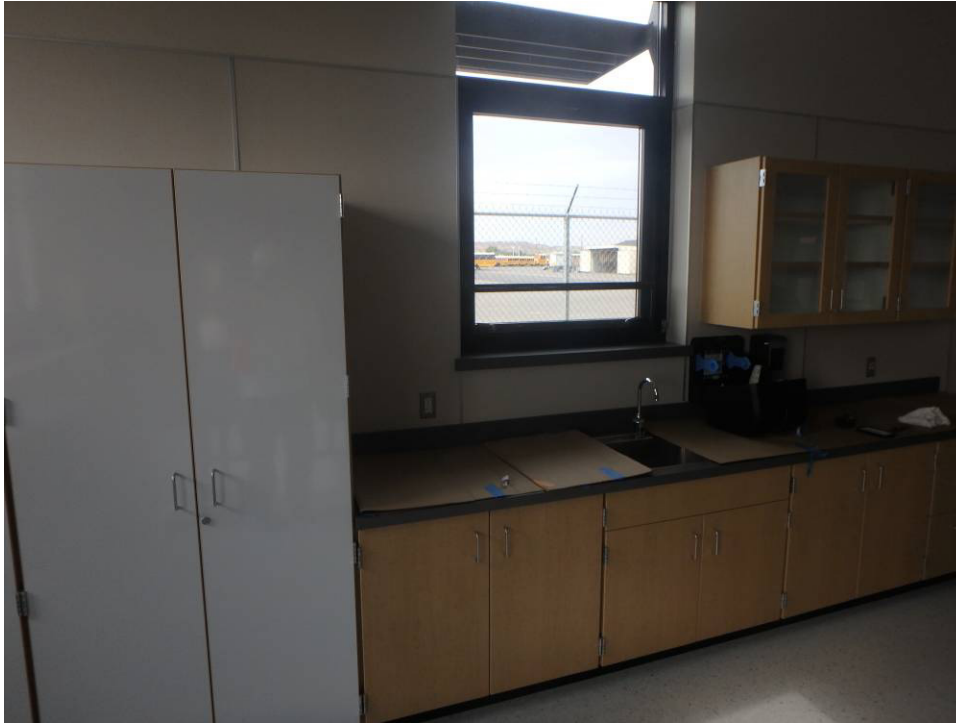
Looking at the casework on the south wall of the south classroom
