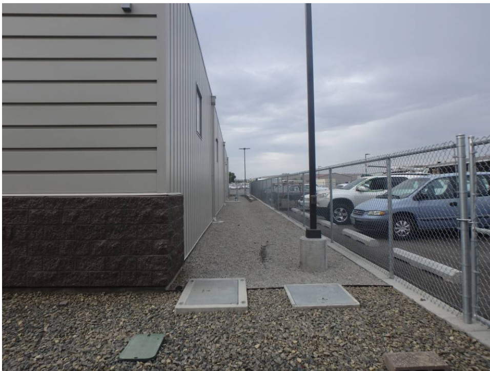
Looking south along the west property line and west elevation
