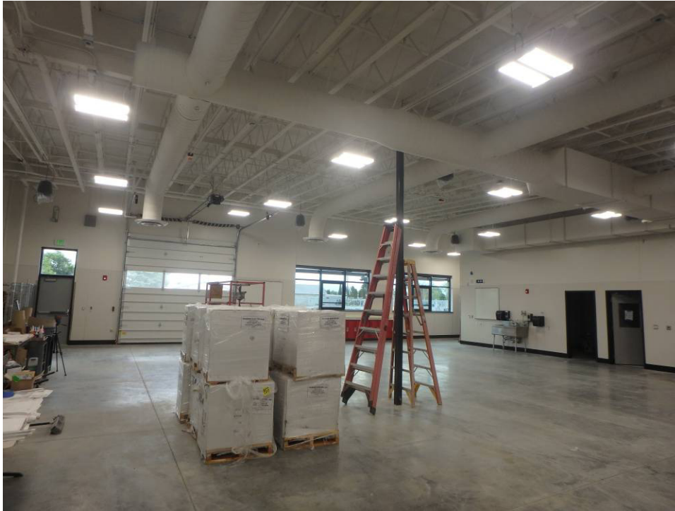
Looking east across the shop towards the east wall
