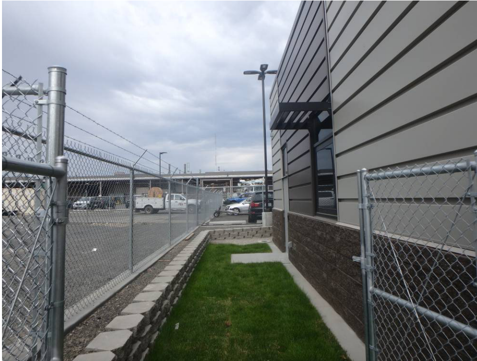
Looking west along the south elevation
