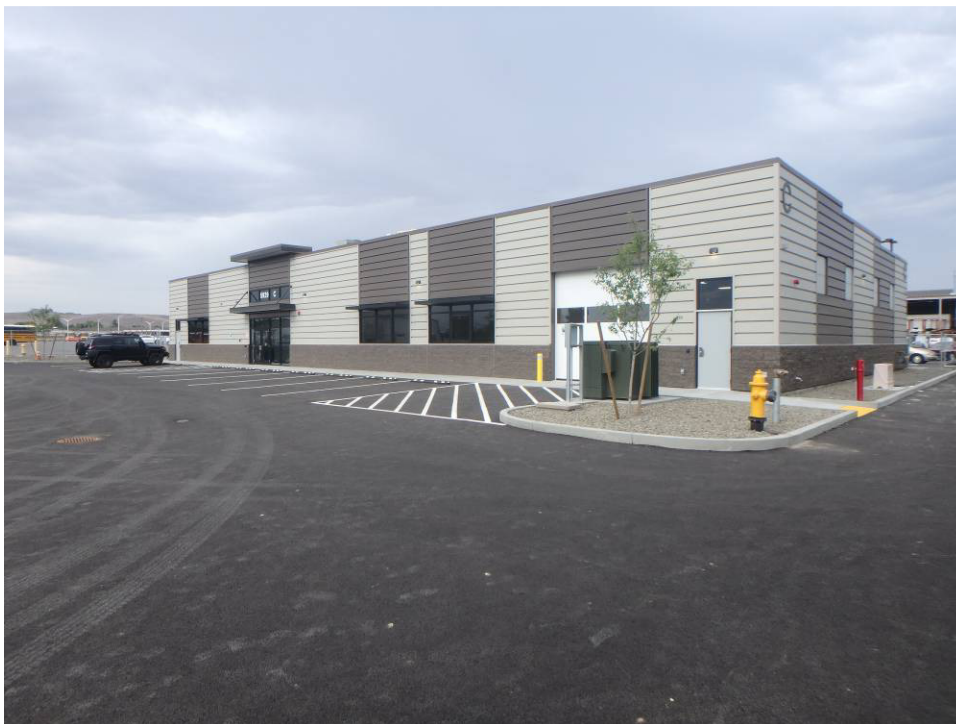
Looking southwest at the East elevation
