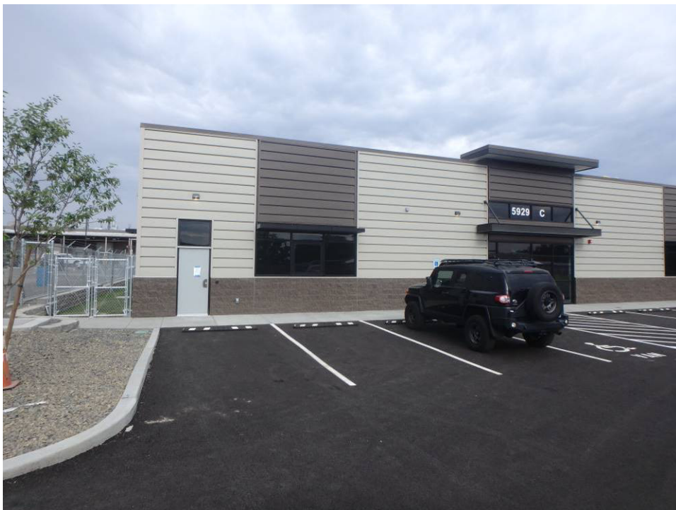
Southeast corner of the building
