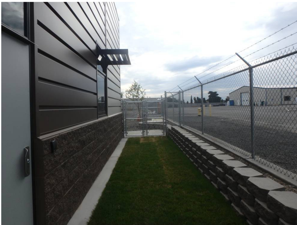
Looking east along the south elevation
