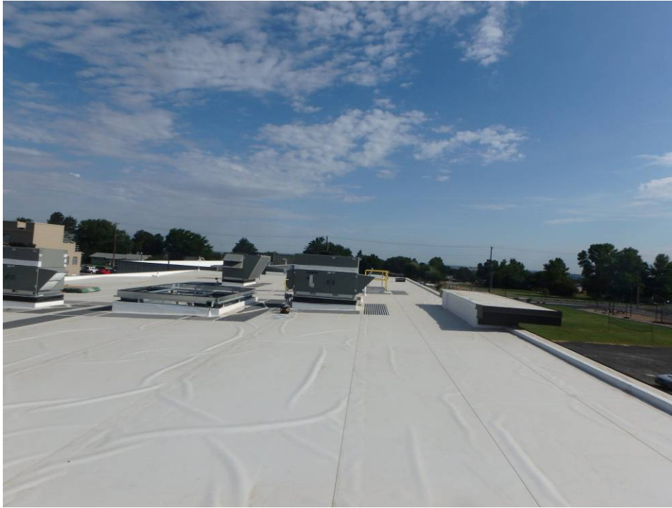
Looking north along the east edge of the building (6/27)
