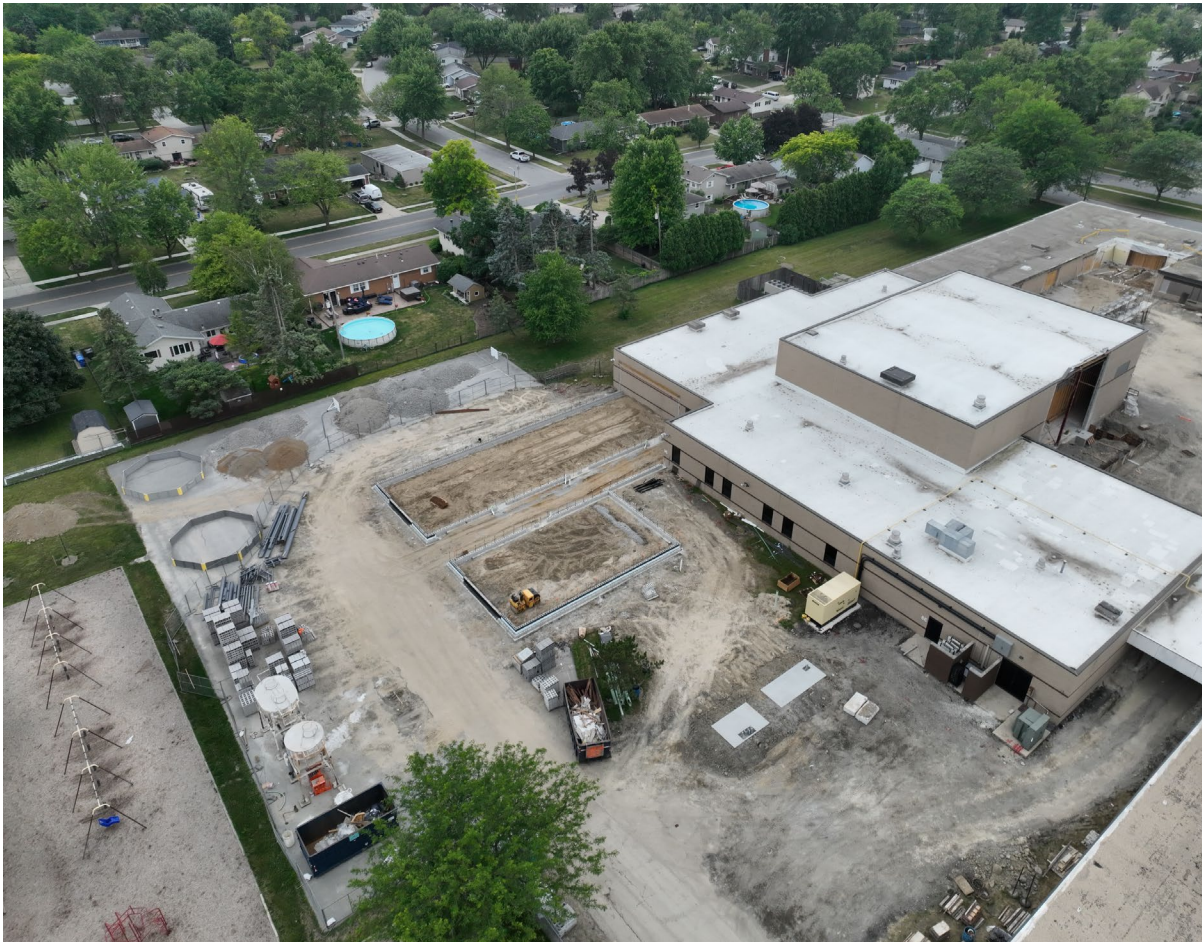
Addition Footings and Prep
