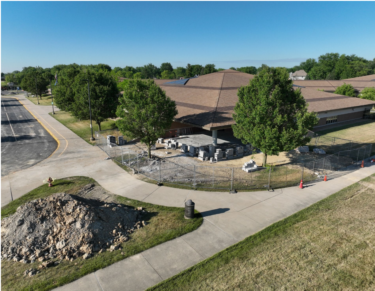
Classroom Renovation Exterior Update
