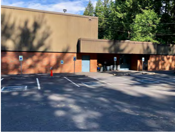
From ADA stalls on side of building, continue to the north for building and/or field access.
