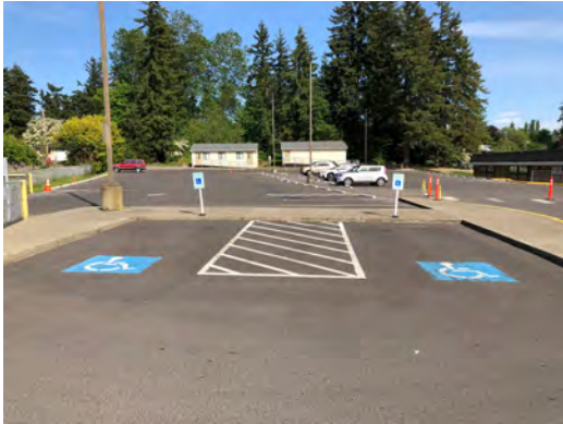
ADA stalls in Mountain View parking lot. Crosswalk to sidewalk missing.
