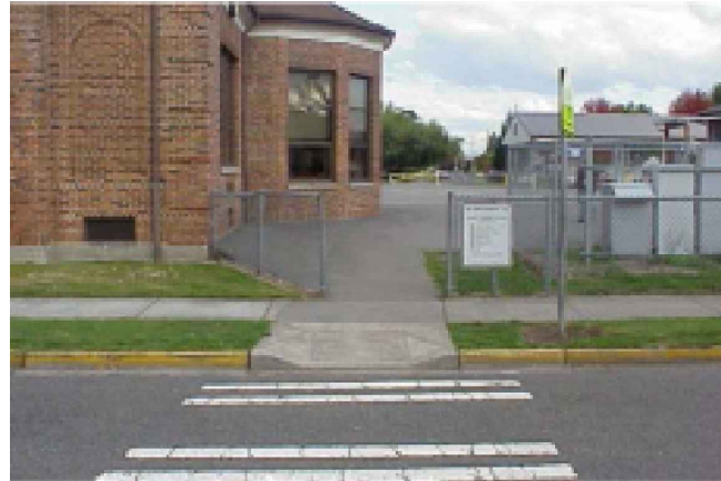
For field access, continue through the gate, and keep right. Note that the curb cut here does not meet all ADA standards.
