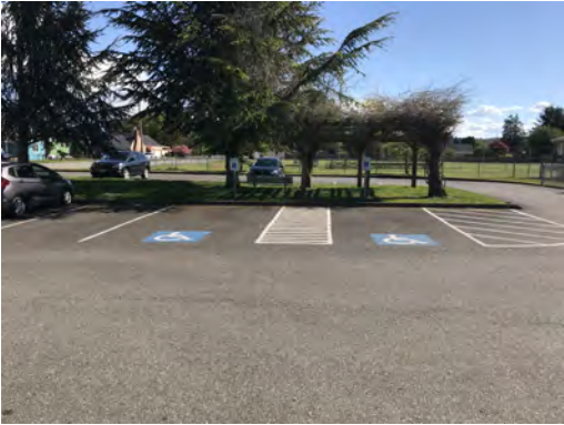
ADA stalls in parking lot. Crosswalk to sidewalk missing.
