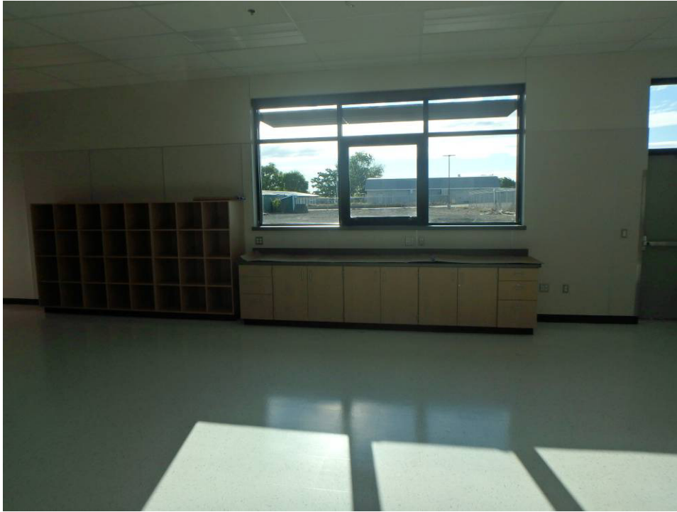
Looking at the casework on the east wall of the south classroom
