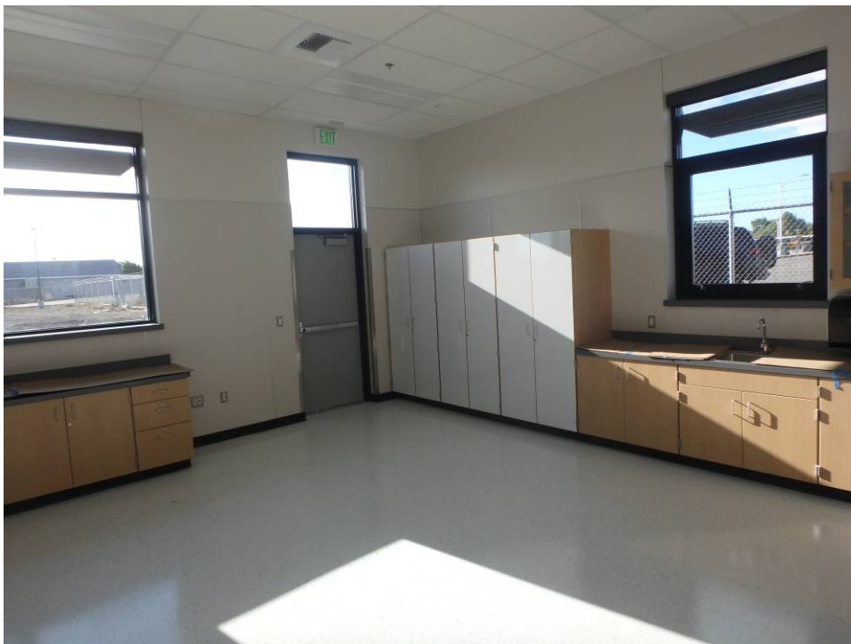
Looking southeast corner of the south classroom
