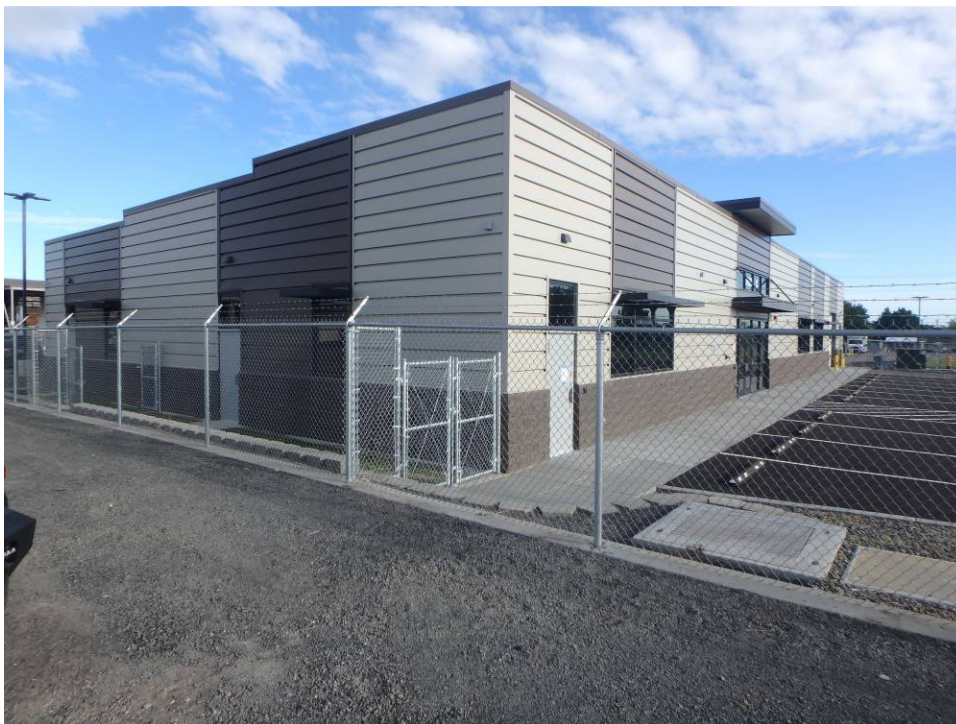
Southeast corner of the building
