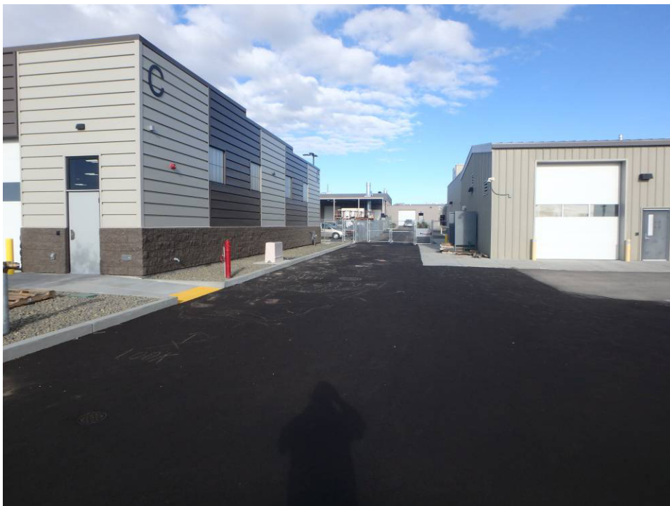
Alleyway – looking west and the North elevation
