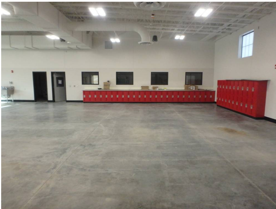
Looking south at the shop's south wall
