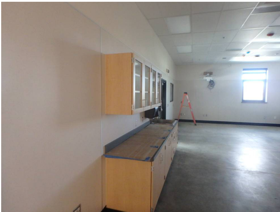
Looking south at the lab casework on east wall
