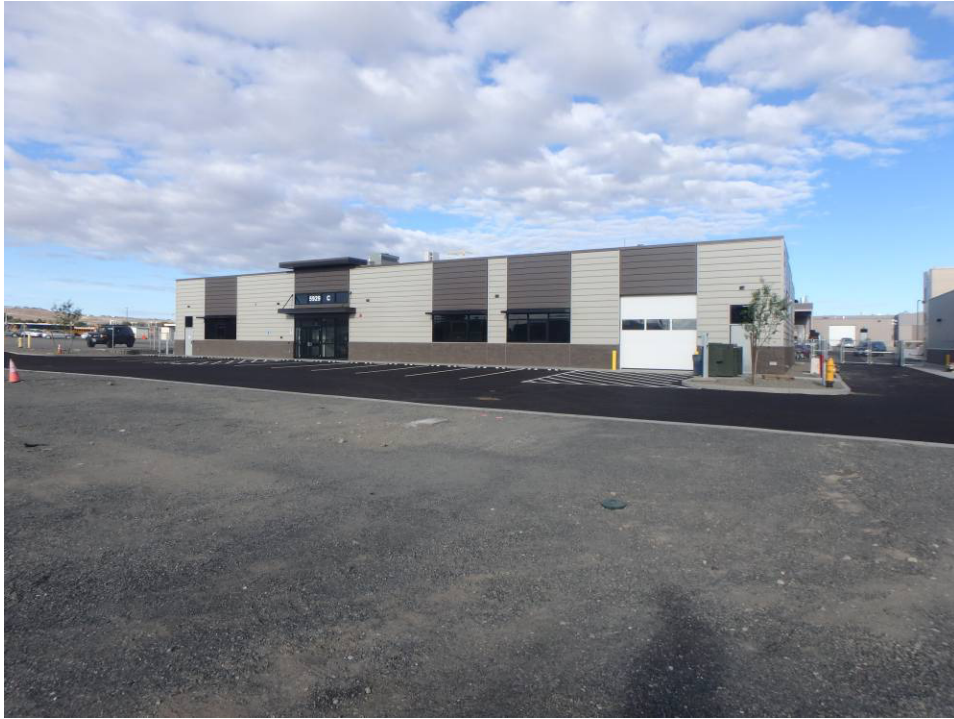
Looking southwest at the East elevation
