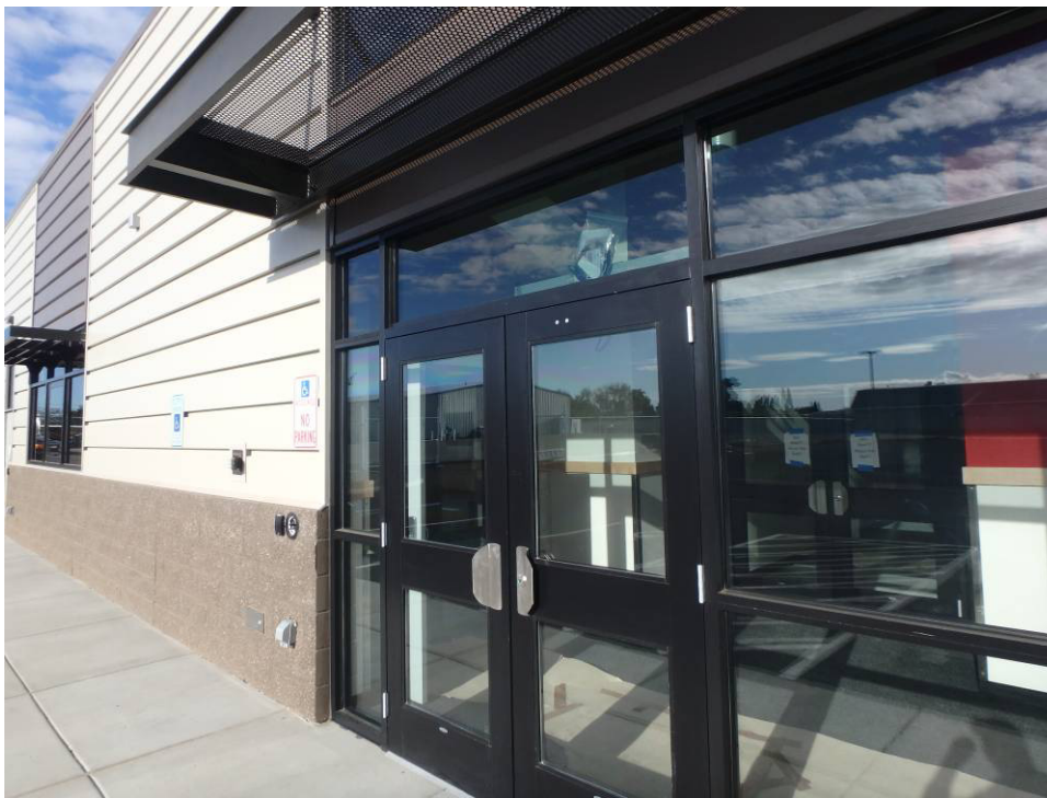
Main entry doors and sidelites
