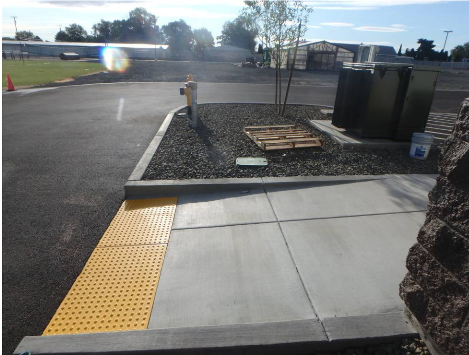
North ramp and peninsula
