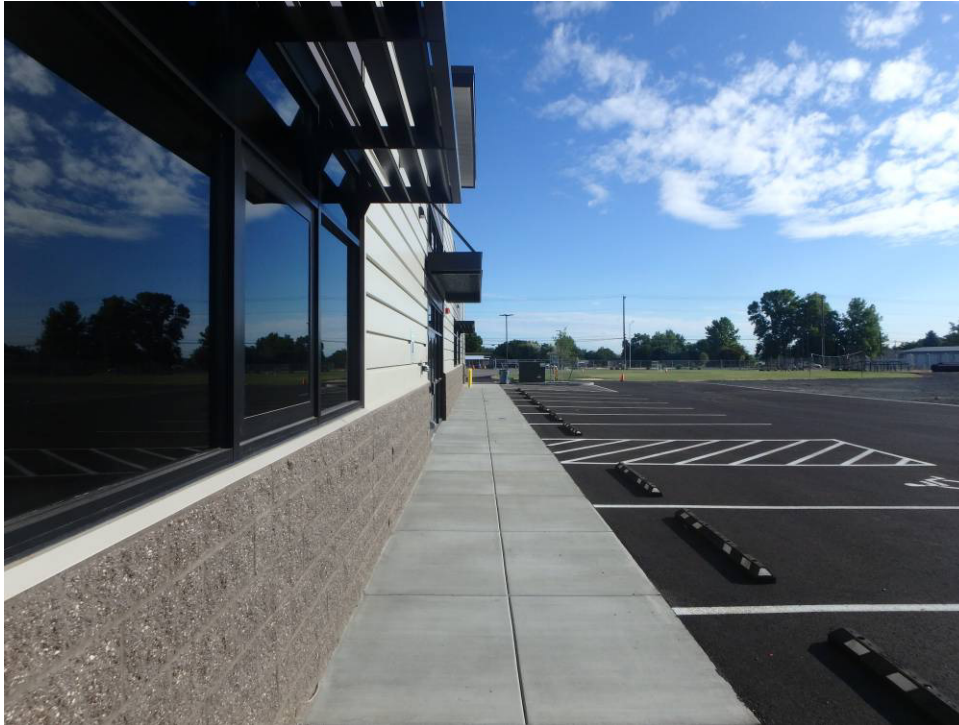
Looking north along the front sidewalk
