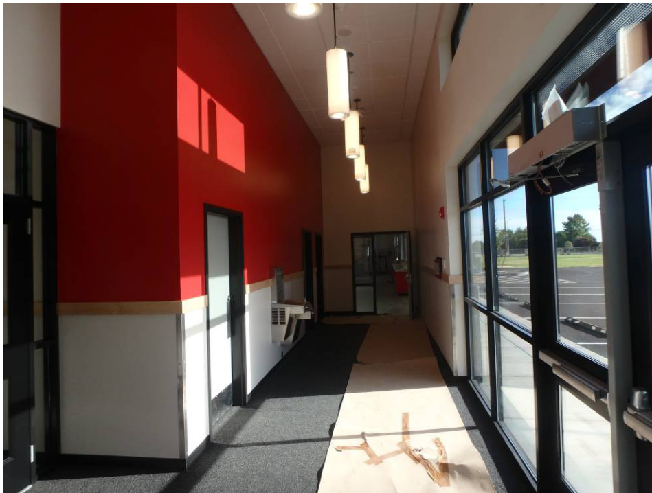
Entry – looking north
