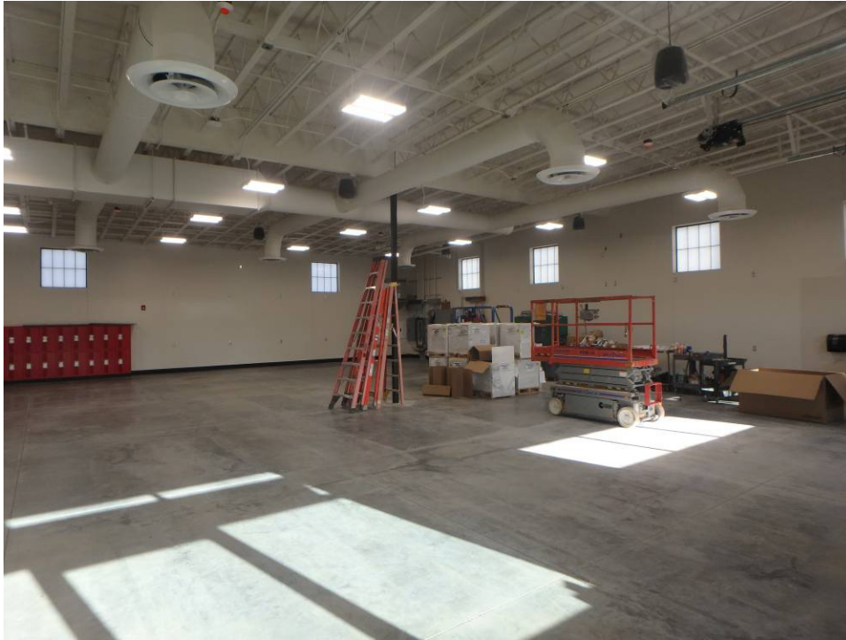
Looking northwest into the shops northwest corner
