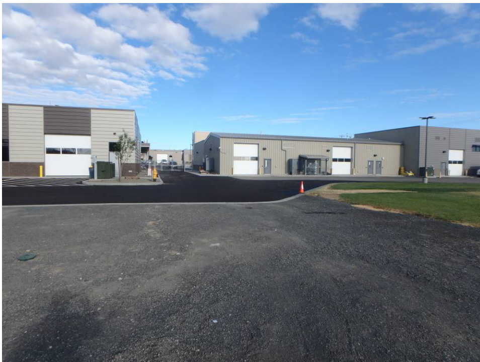
Looking at the north end of the East elevation and the alleyway and TTE
