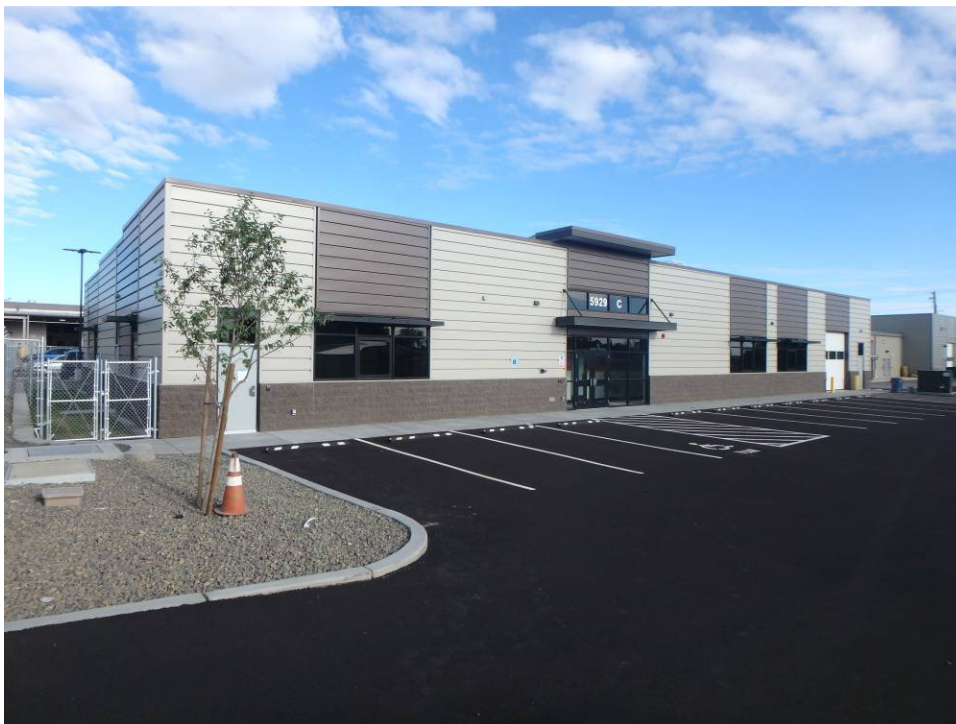
Looking northwest at the East elevation
