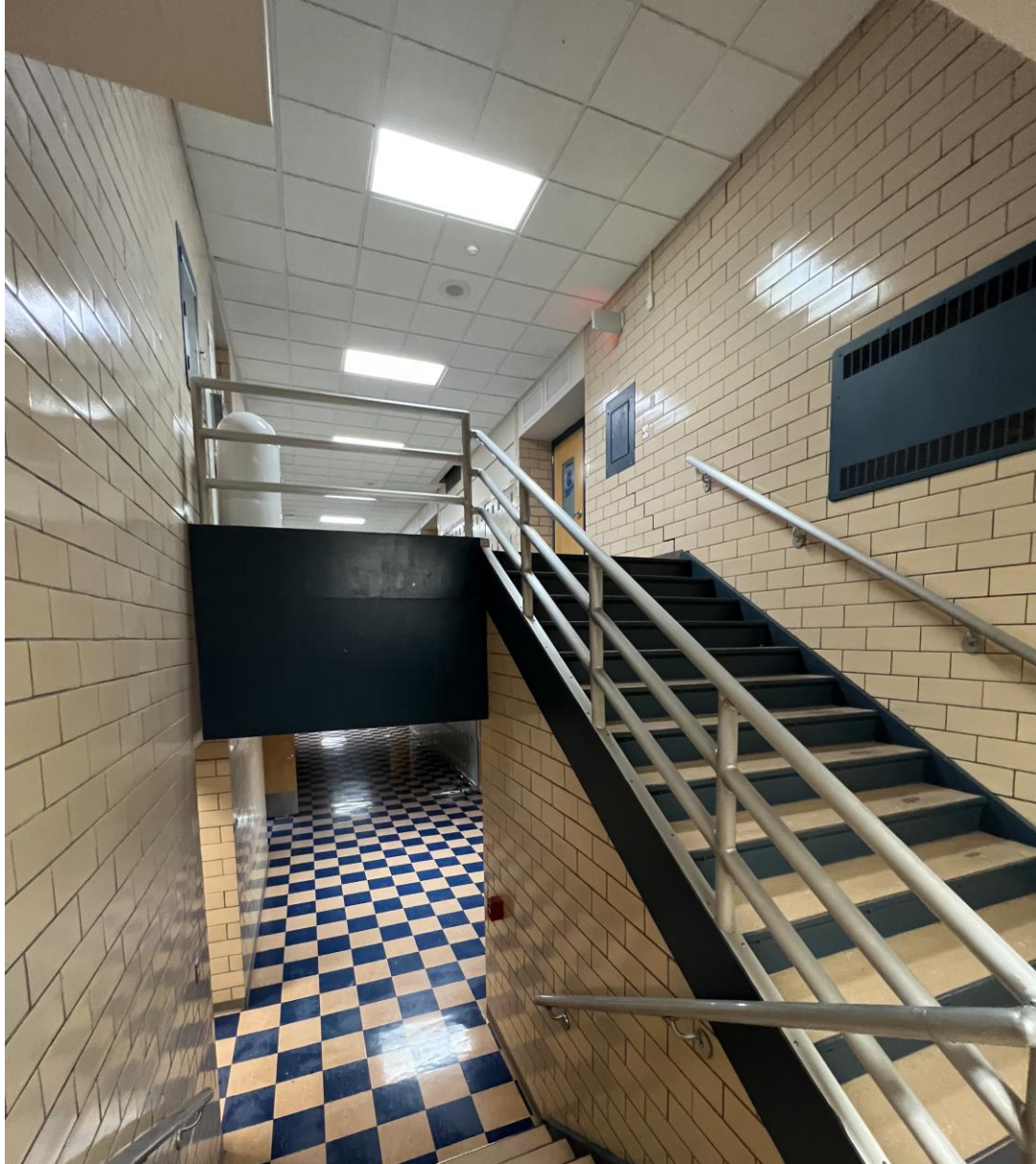
Stairwell lacking separate handrail from the guardrail and the spaces between the railings exceed the maximum 4 inches.
