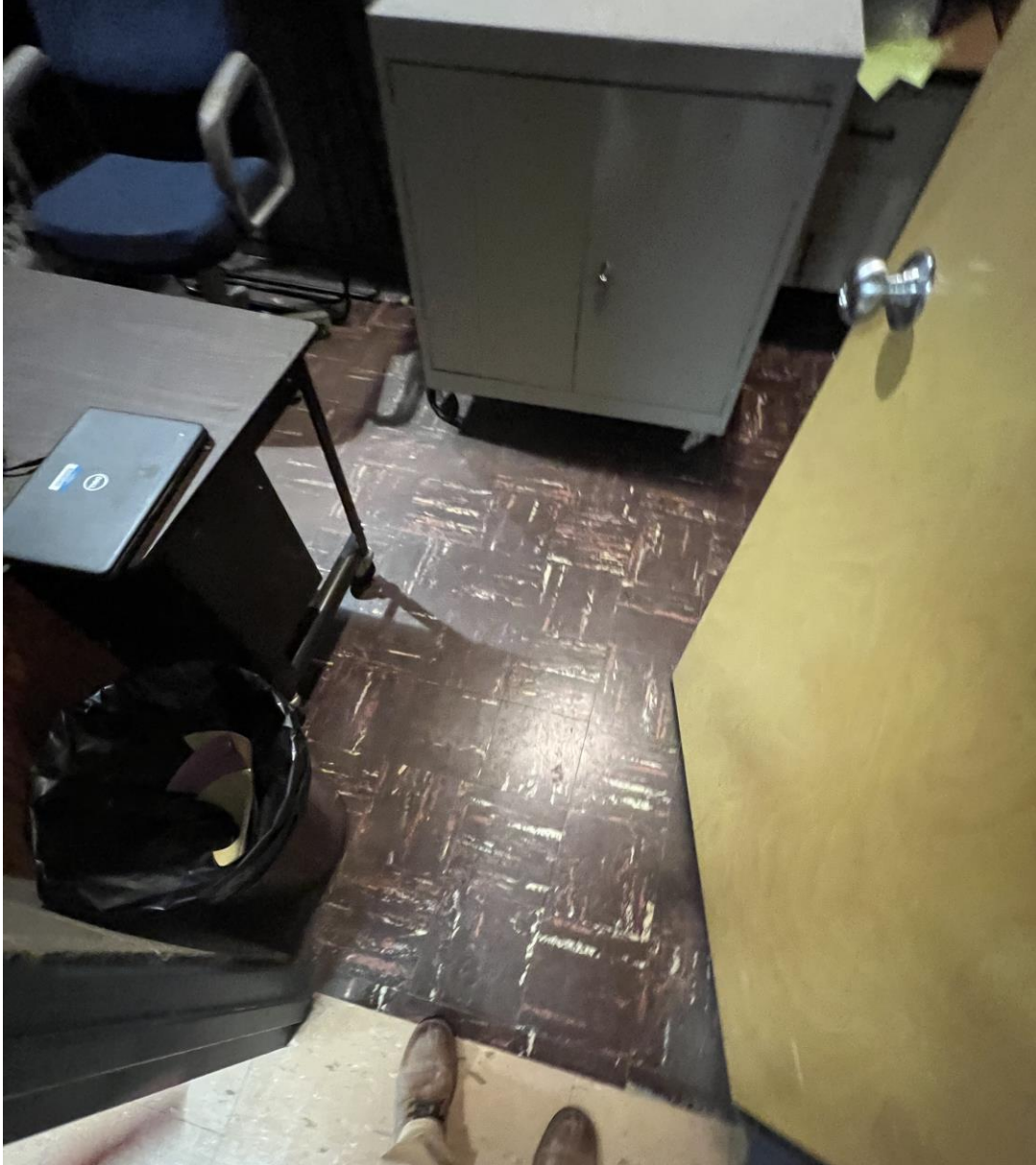
Original tile throughout the school that has reached its end of life.
