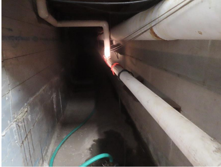
Figure 3: Tunnel near classroom #2
