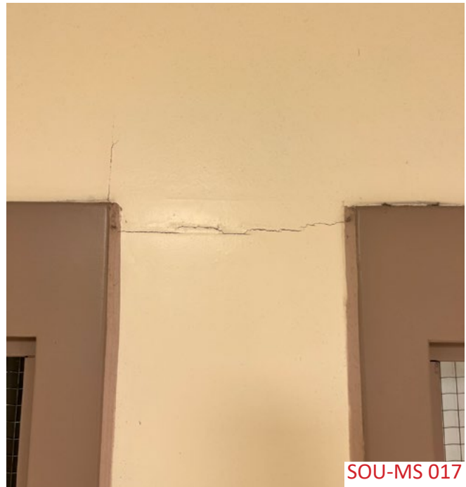
There is horizontal cracking on the dry wall between many of the interior doors.
