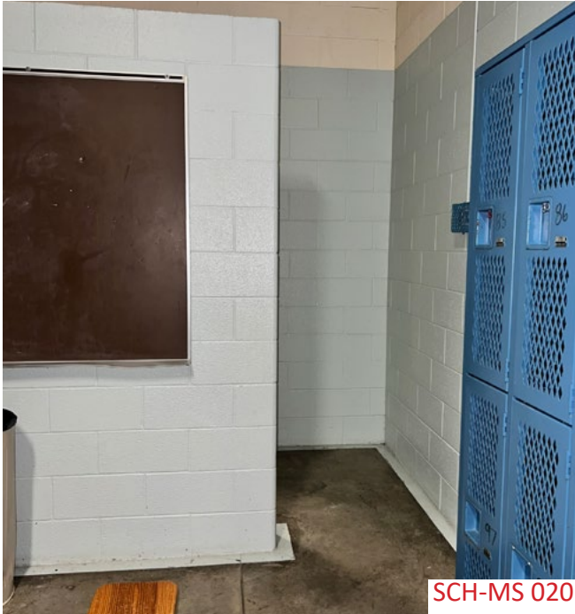
Entry into locker rooms do not have adequate clearances for accessibility
