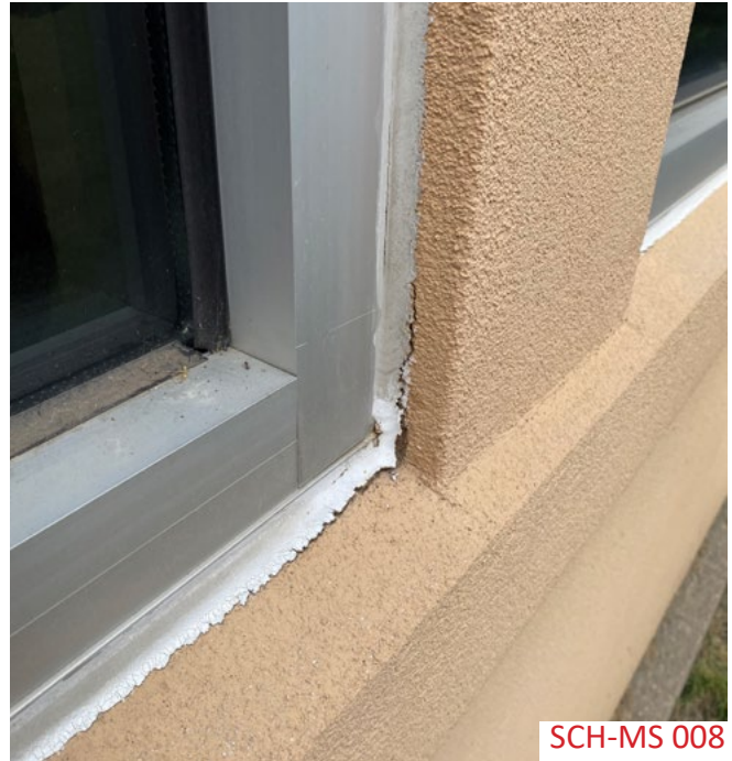
Caulking is worn and should be replaced as well.
