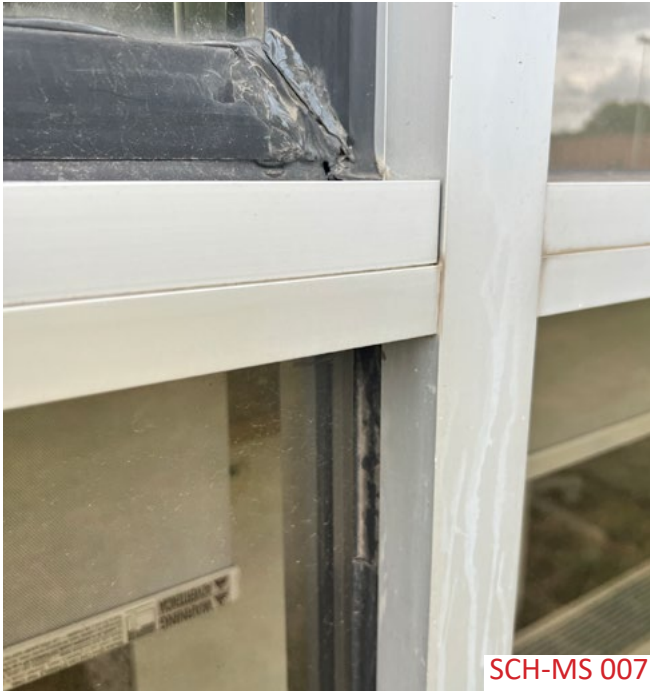
Window gaskets are deteriorating and need to be replaced.
