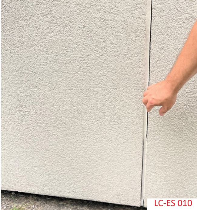
Caulking should be redone as it is worn and deteriorating.
