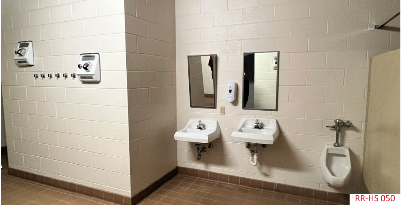
All three men's locker rooms are missing a lower urinal.
