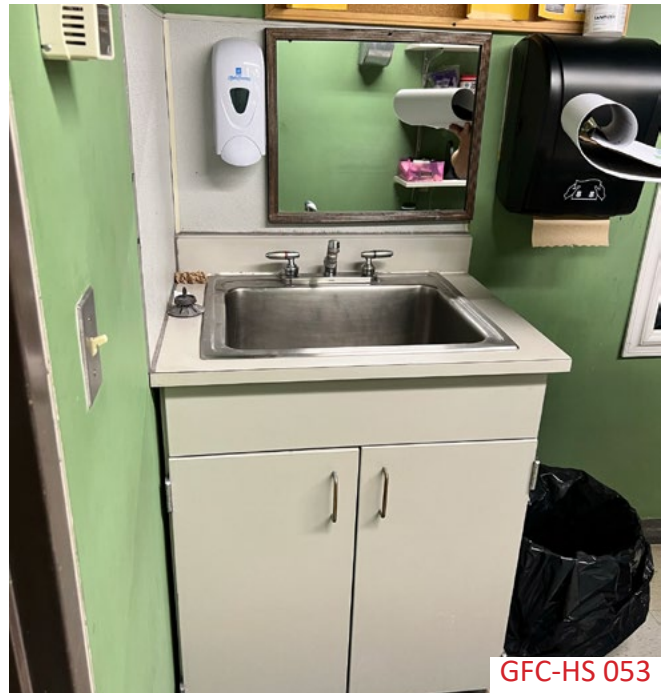
Sinks in all the dressing rooms are not accessible.
