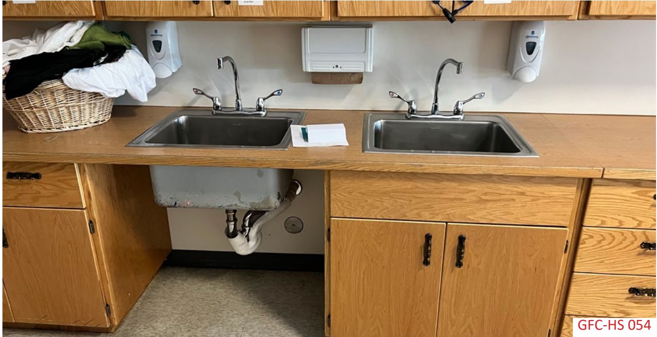
Art classrooms (Rooms 102 and 103) lack an accessible work area and the sinks do not have enough clearance underneath to comply with ADA standards.
