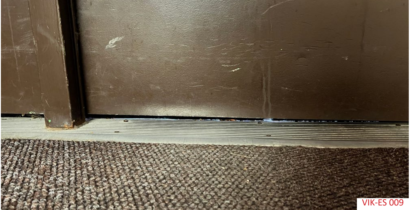
Weather stripping could be replaced.
