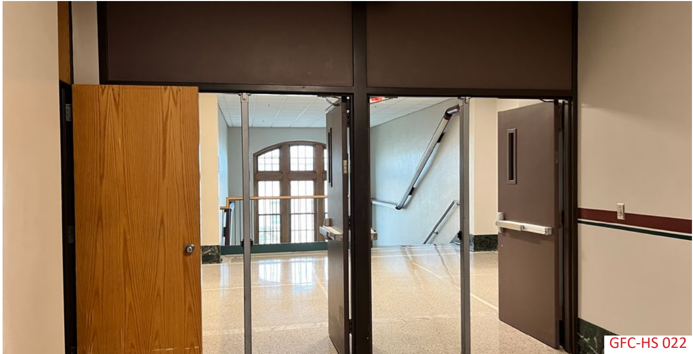
The corridor partition doors with a mullion do not allow sufficient clearance for wheelchairs.
