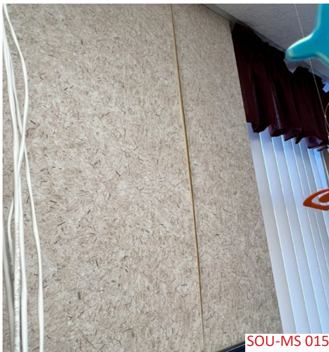
There are several areas where the vinyl wall covering is releasing from the gypsum substrate.
