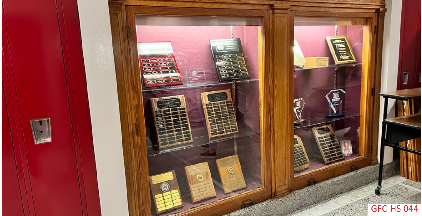
Display cases throughout the school do not have required safety glass.
