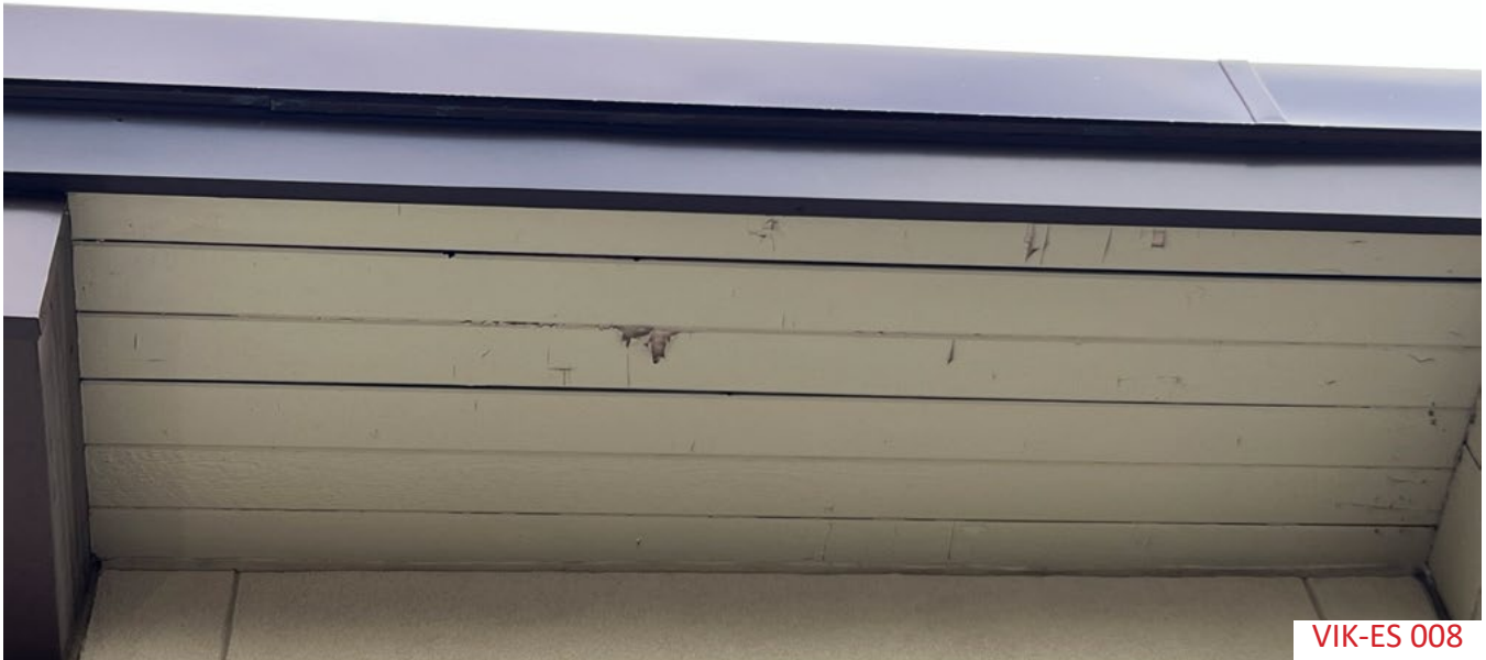
In areas of overhangs around the building, paint is peeling underneath the wood.
