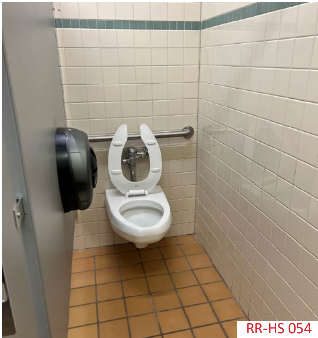
Many restrooms in the building are not accessible. Most restrooms where a larger stall is present do not meet clearance requirements for accessibility.
