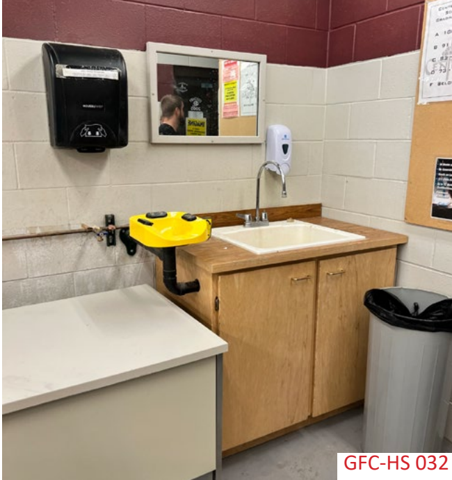
Woodshop has no ADA compliant workstations, no accessible sinks, and no accessible eyewash station.
