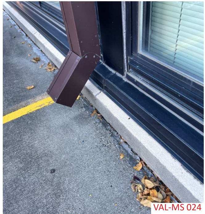
Overall, the windows appear to be in good condition but the sealant and gasketing within the windows are in poor shape and need to be redone.
