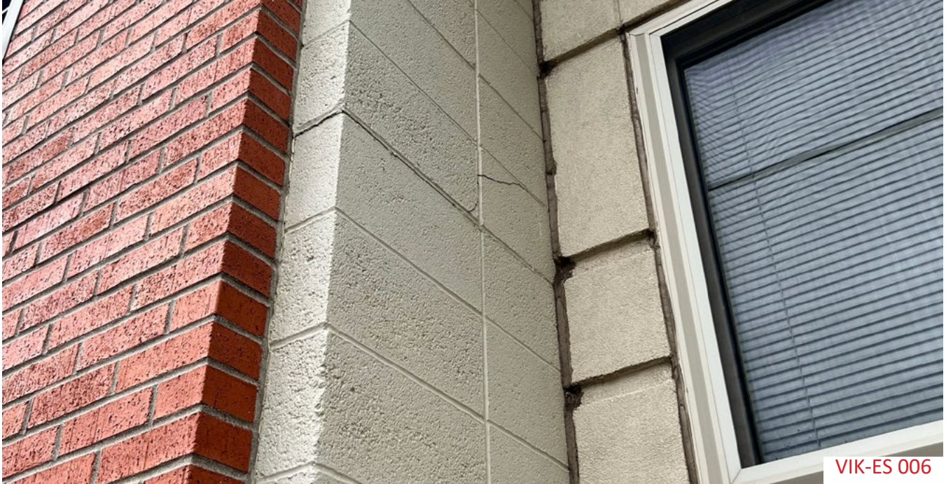
There is some cracking on exterior CMU brick.
