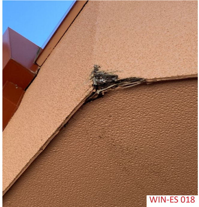
The plastered wood over the entrance is showing signs of age and is deteriorating.
