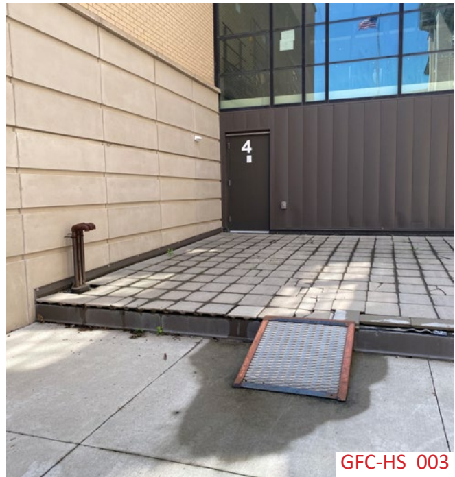
On the outside of door 4, pavers are worn and cracked, exposing the roof and the space below.
