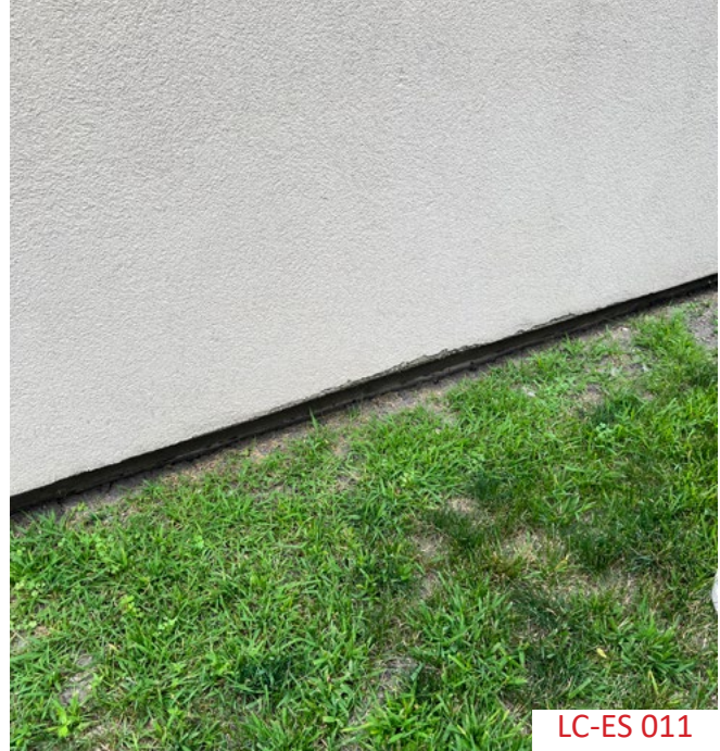
There is damage to the bottom edge of the EIFS around the perimeter.
