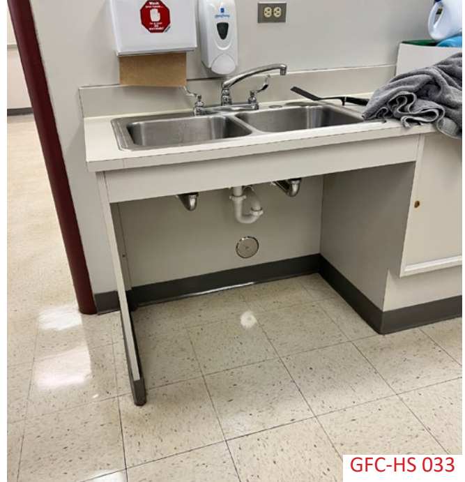
The pipes underneath the accessible sink in Room 24 are not protected.
