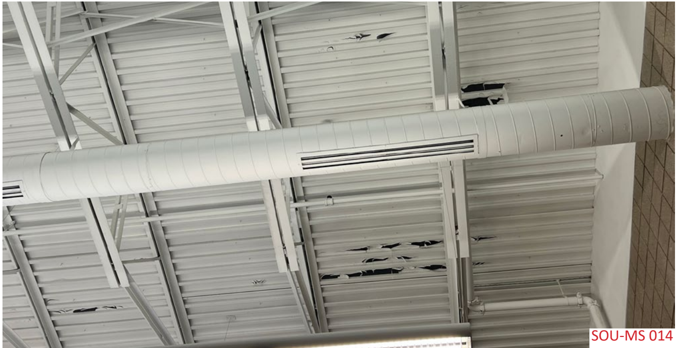
Another area of concern with ceiling is in the library where there is paint flaking from the steel deck paneling.
