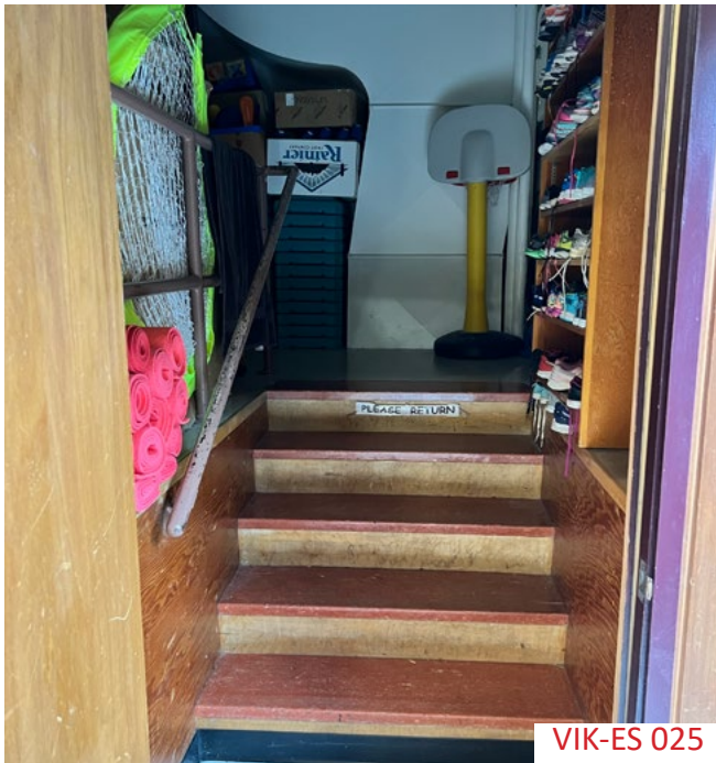
Stairwells leading up to the stage do not have handrails on both sides.
