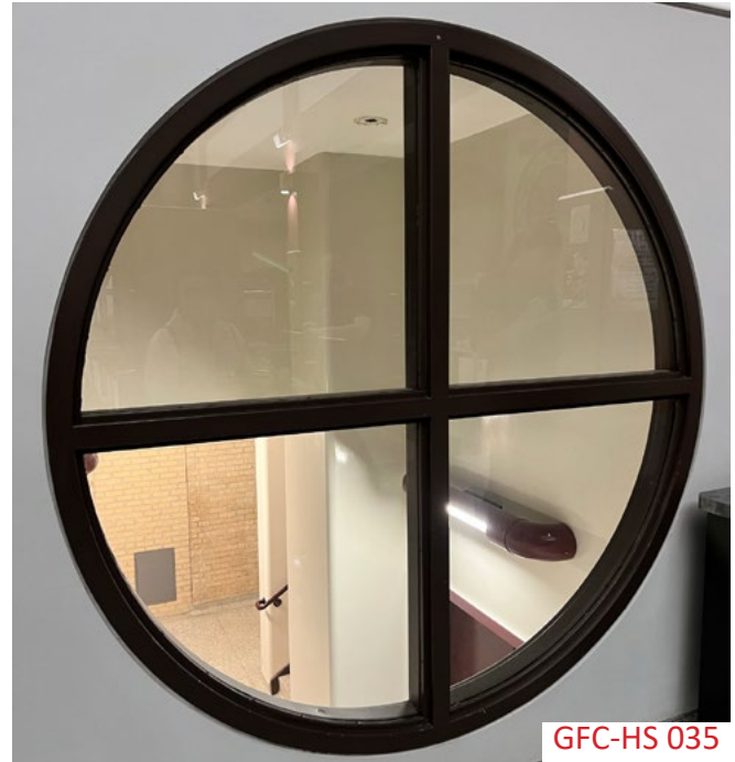
Interior windows in the commons/cafeteria that face the adjacent stairwell do not have the required safety glass.
