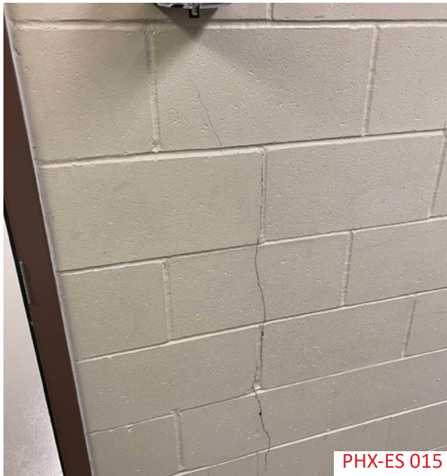
There is cracking in a CMU wall adjacent to a steel column that can be seen from the mechanical room and the hallway.
