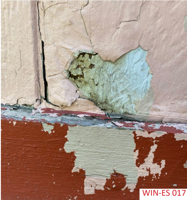
The paint is peeling off as well, further reducing the water protection of the exterior.
