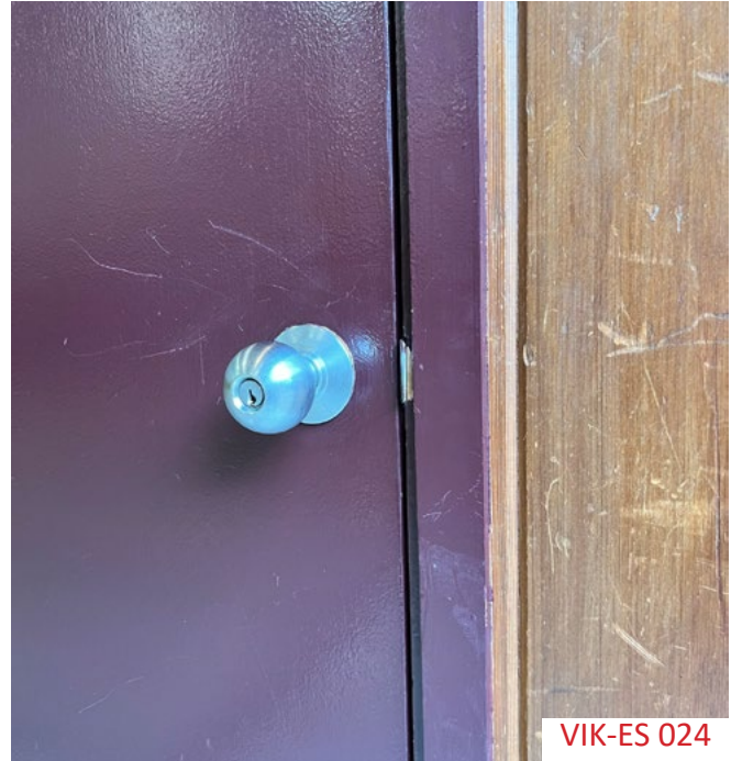
Doors in STAR rooms and storage rooms in the gym do not have accessible door hardware.
