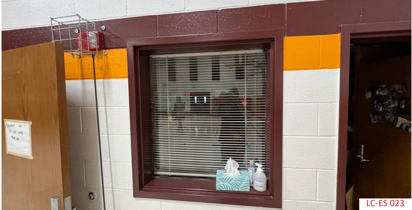
Window in the gym does not have the required safety glass
