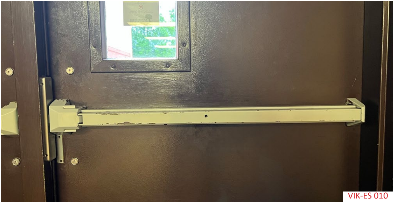
Weather stripping could be replaced and potentially door hardware.
