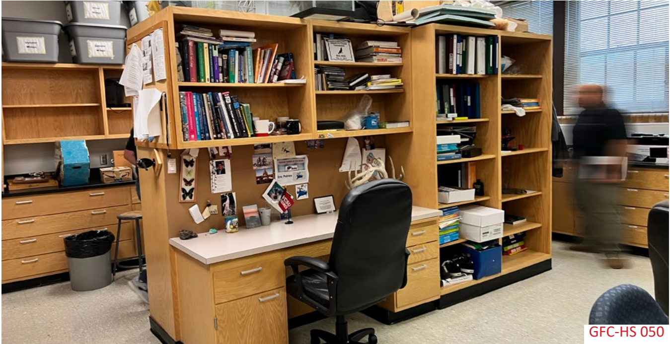
Casework within the biology office (Room 306) lacks sufficient clearances for accessibility.
