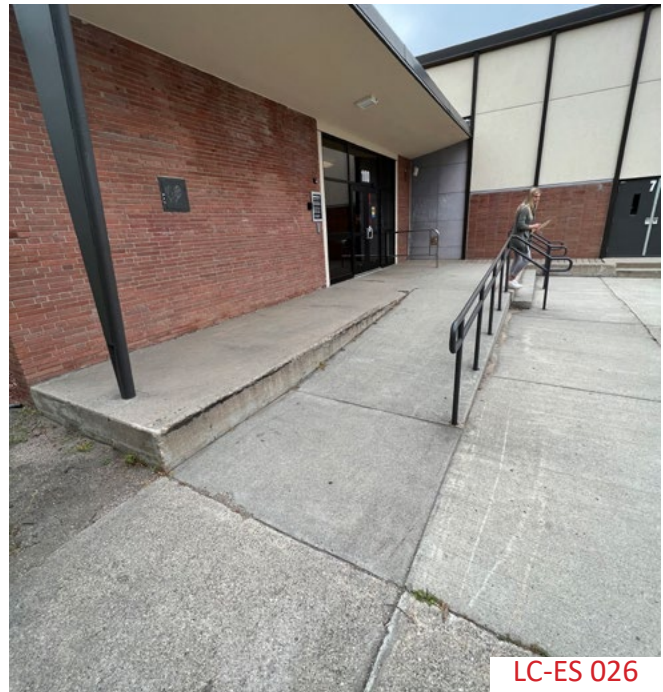
Ramp outside of Door 1 is missing a railing as required by code
