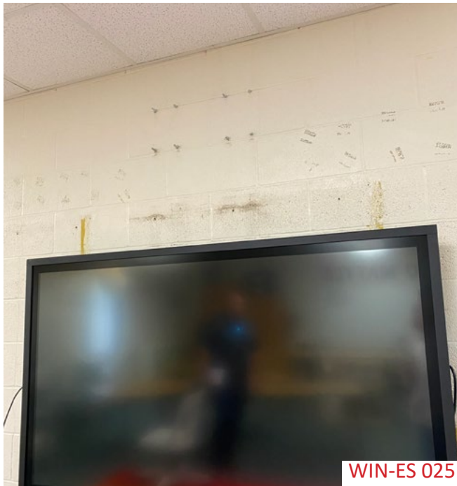
In Room 147C, the CMU paint has patches and could use some retouching.
