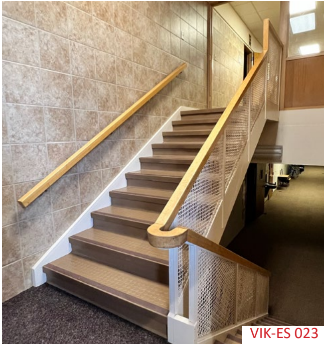
Handrail cross sections exceed size limitations per code.
