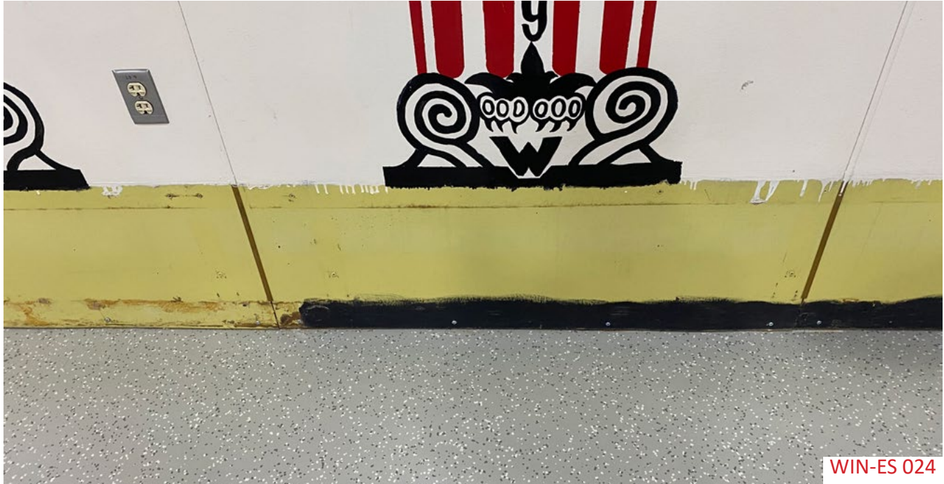
A gypsum board wall in the gymnasium needs painting after an attached bench was removed.
