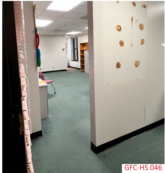
The walls in the offices in Rooms 228 and 317 do not allow sufficient clearances for accessibility.
