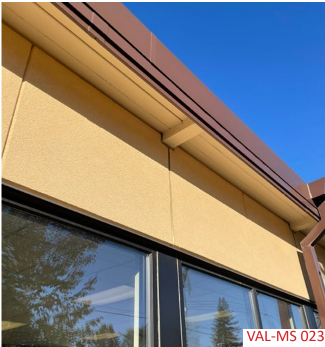
There are gaps in the soffit that need to be addressed.
