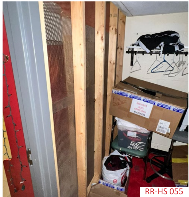
There is exposed wood structure in the storage area in the physical education office that is combustible and should be covered for fire safety.
