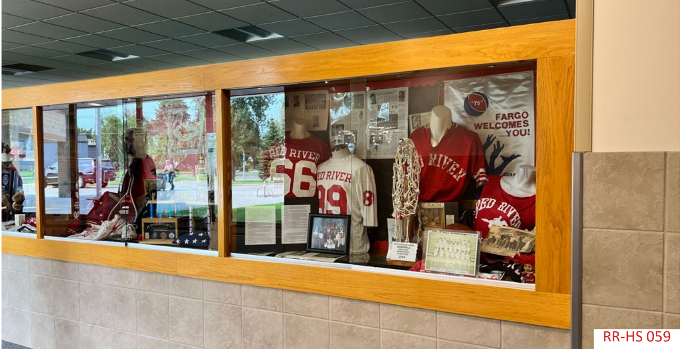
Display cases throughout do not have required safety glass.
