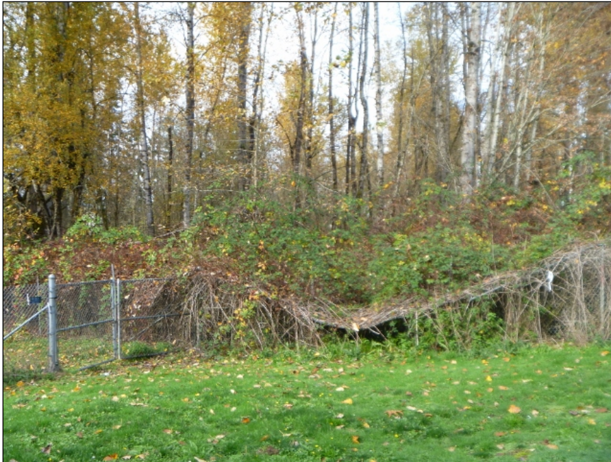
Photo 3. NGPA Fence damaged or failing in a few locations.
