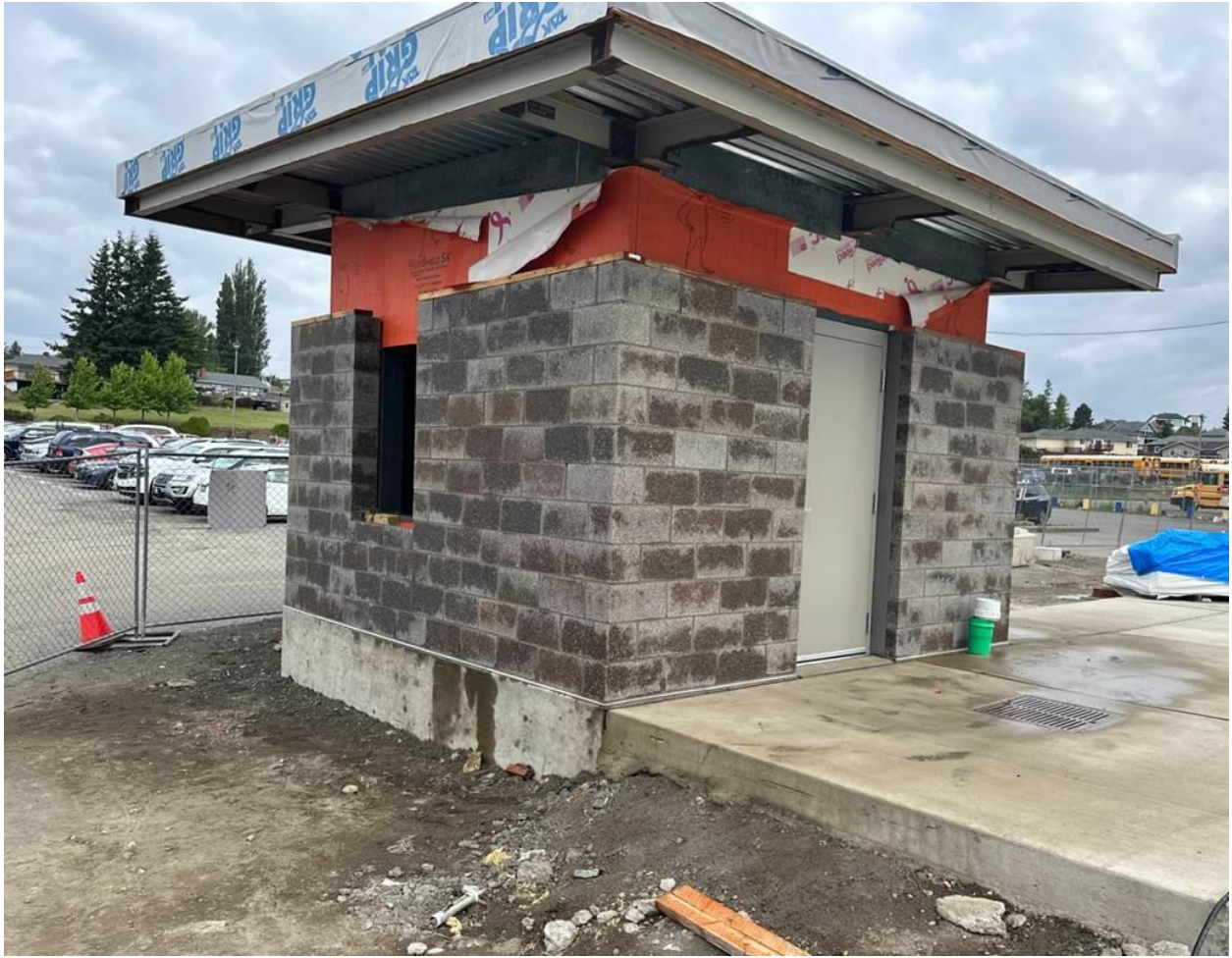
The masonry at the new Athletic Field ticket booth is complete and ready for final finishes
