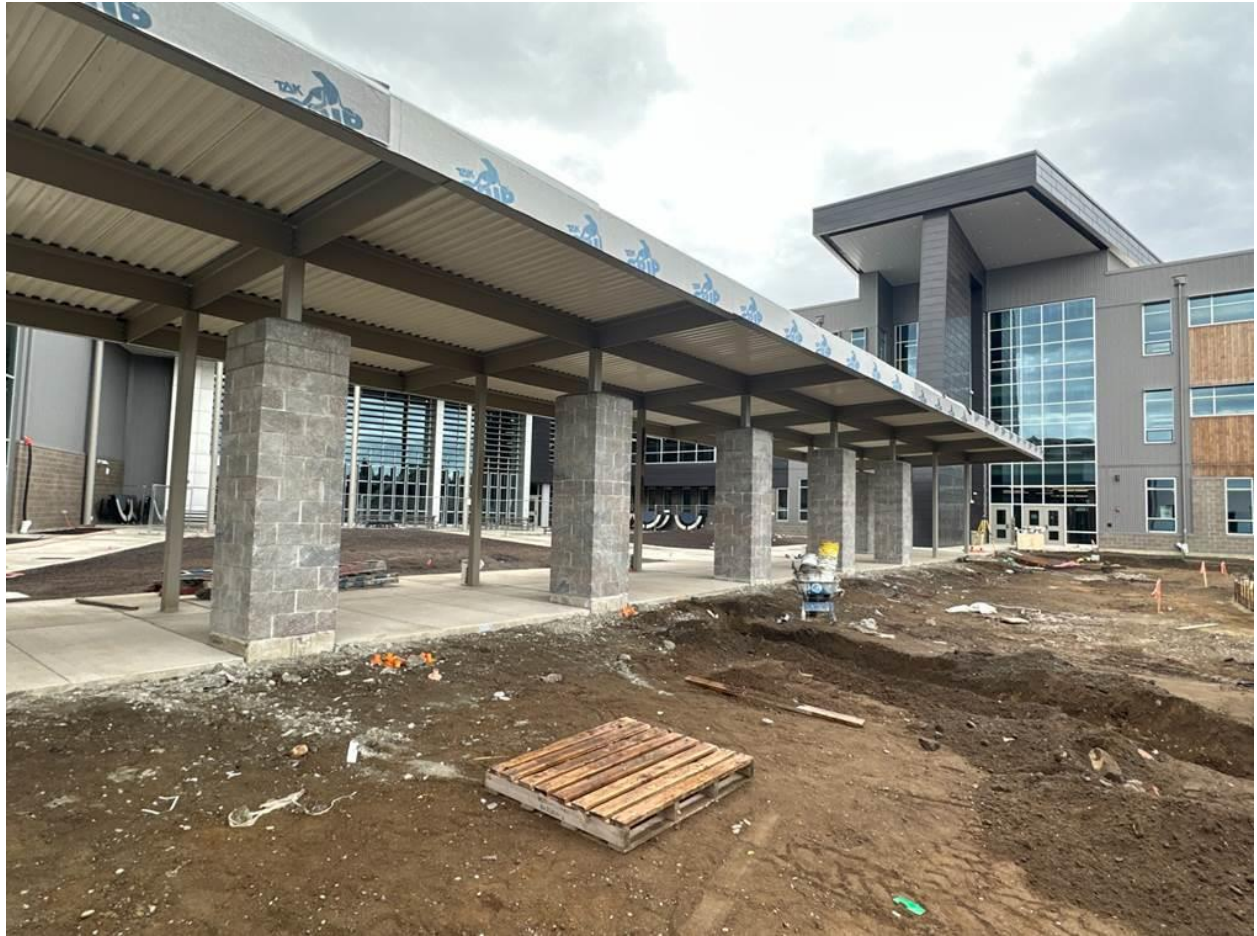
Masonry column wraps in the courtyard area are complete and ready for decorative fencing
