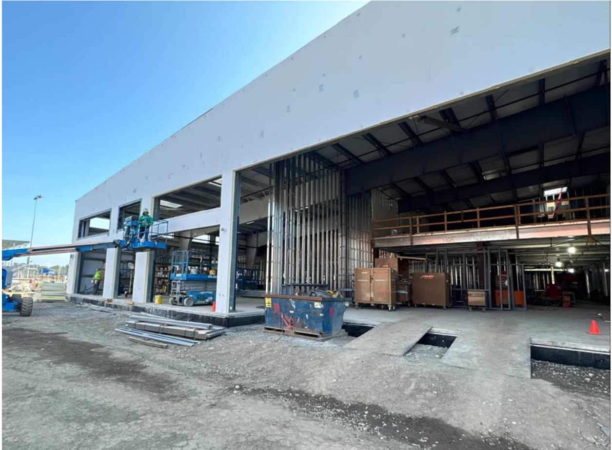
Exterior wall sheathing, framing and the mechanical mezzanine are completed for the CTE Wing
