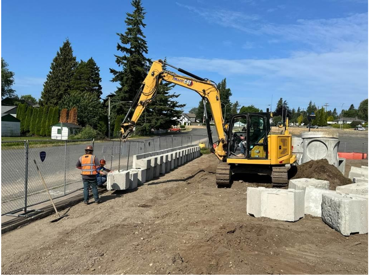
Retaining wall construction at the south end of the new parking area
