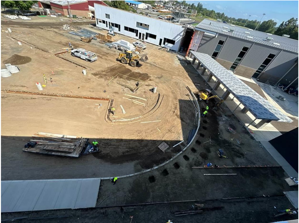
The new parent drop-off loop receiving curbs and gutters in preparation for asphalt
