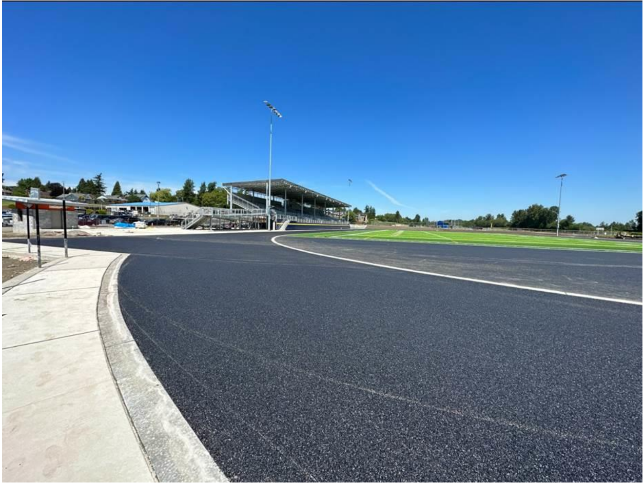
Asphalt installed on the track
