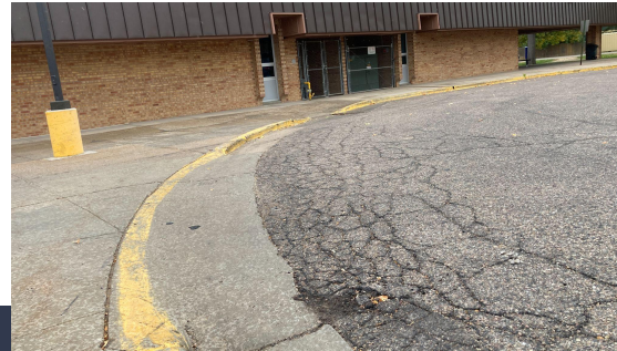
Poor asphalt condition, site drainage issues.
