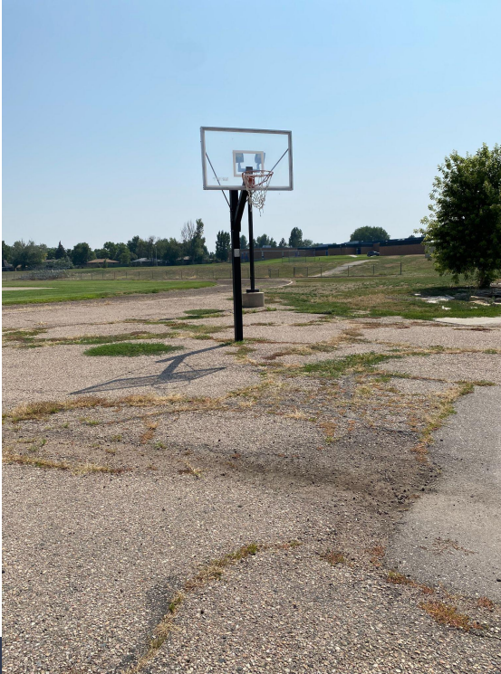
Play pad old, cracking, and deteriorating.
