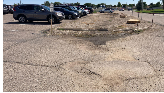
Drainage and paving, area ponding and ices up.
