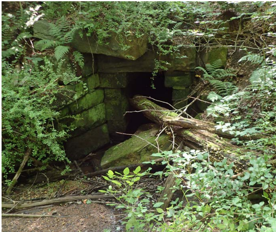
Photo 22: West Elevation Showing Southwest Wingwall Failure
