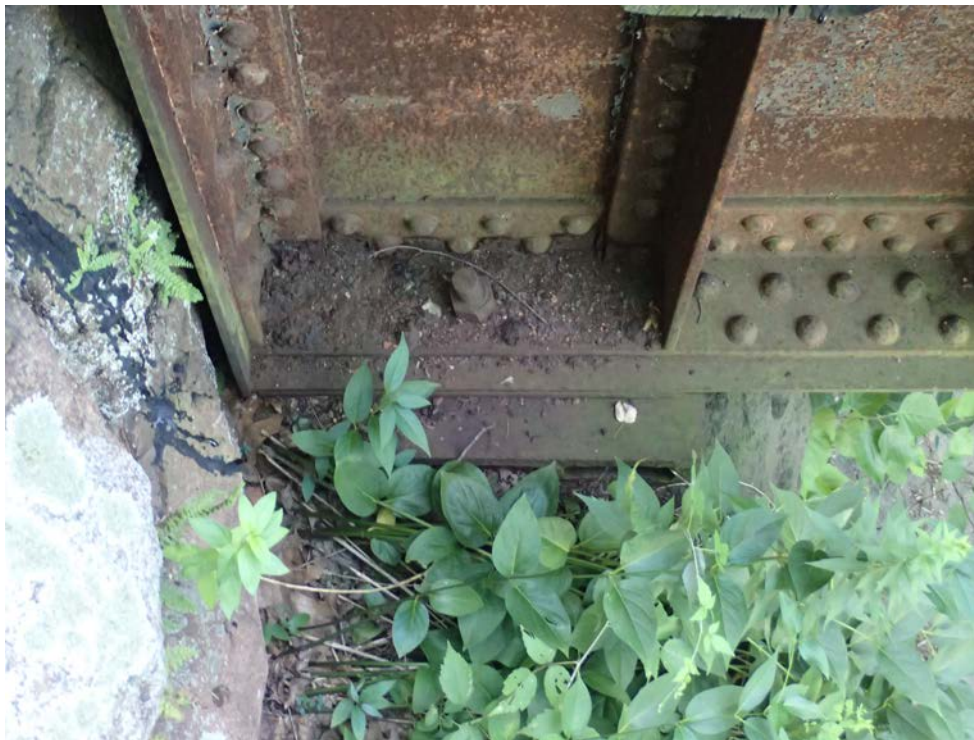
Photo 14: Tipped anchor bolt on the north abutment
