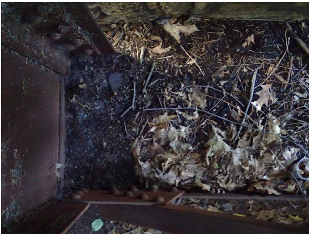
Photo 6: Heavy debris on bearing
