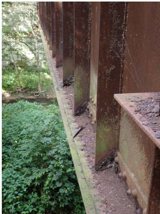
Photo 10: Rusting and deterioration of the steel stiffeners
