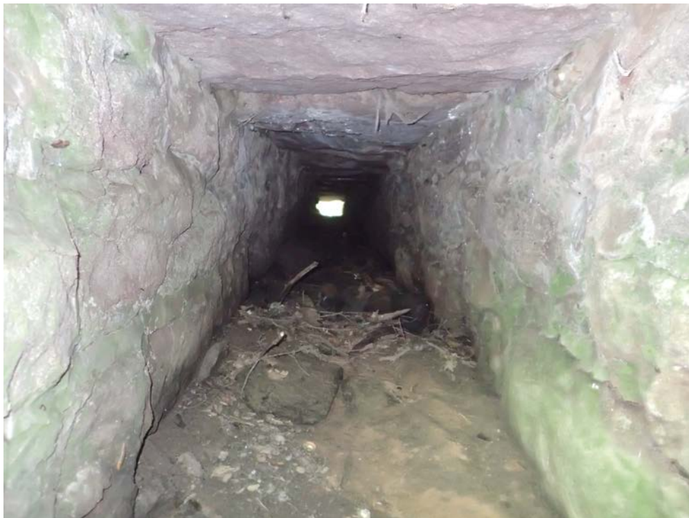
Photo 48: Interior of Culvert 10 with Void in Ceiling
