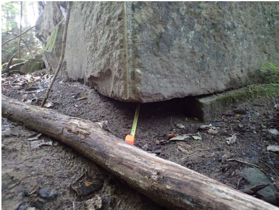
Photo 8: Undermining of center pier
