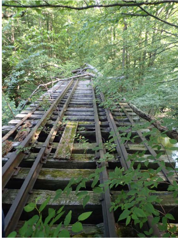
Photo 7: Existing timber deck with railroad ties
