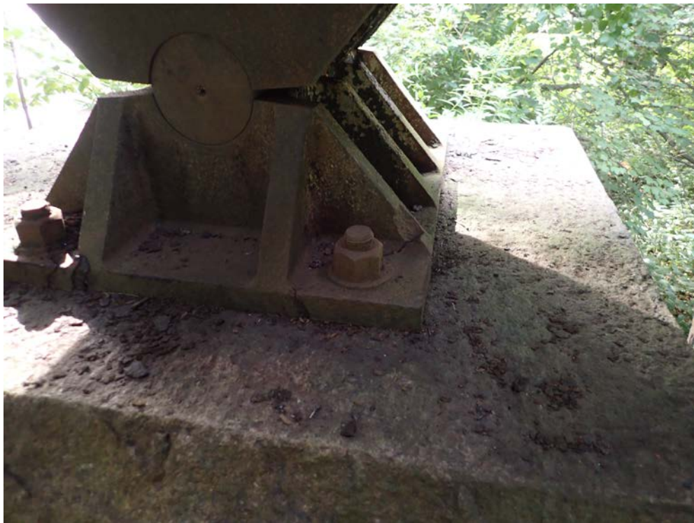
Photo 12: Cracked bearing on the bridge pier
