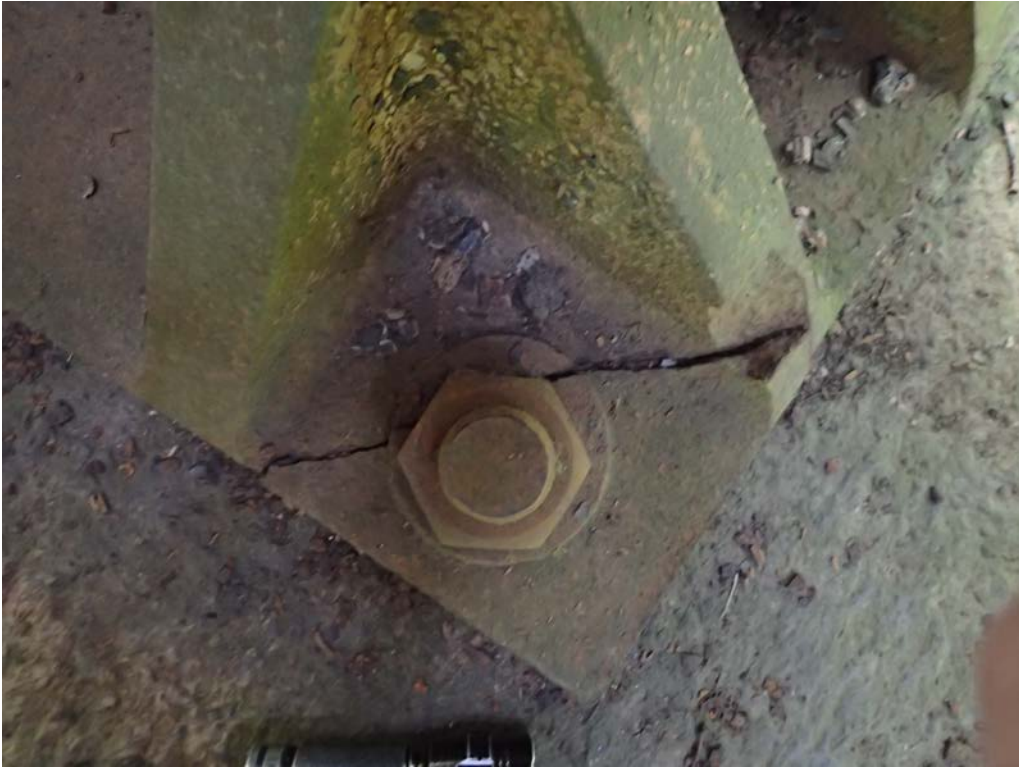
Photo 13: Cracked bearing on the bridge pier
