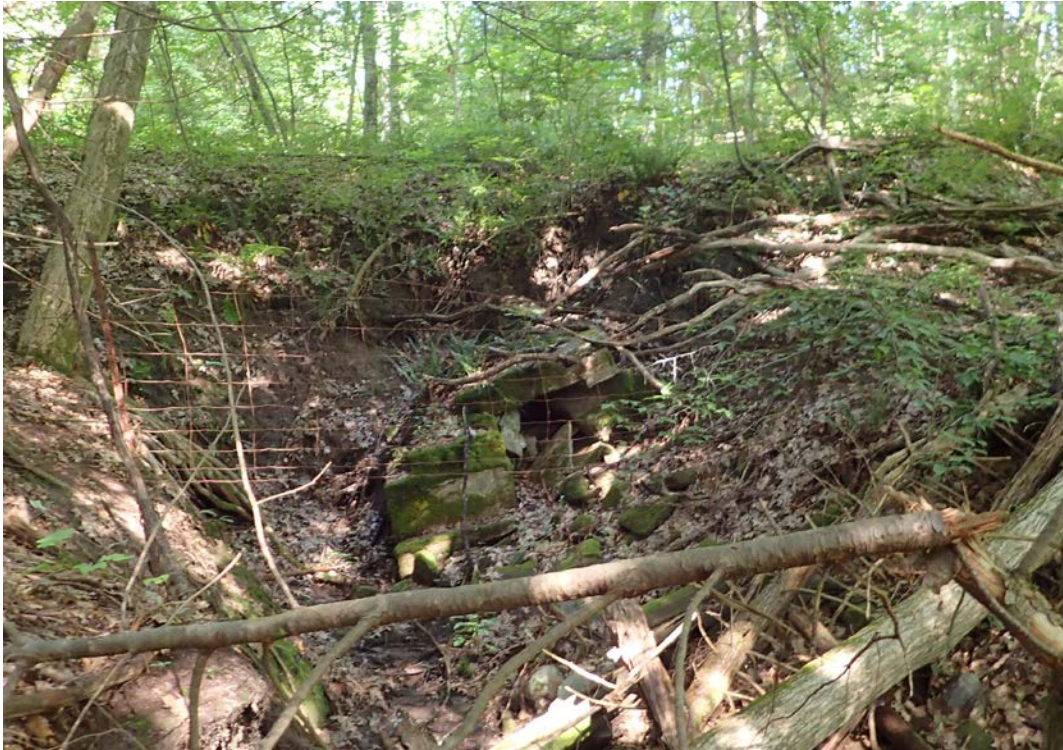
Photo 17: East Elevation showing Collapsed Section
