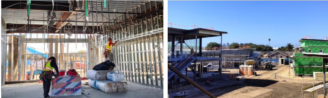
Rose Avenue Elementary School Construction Progress
