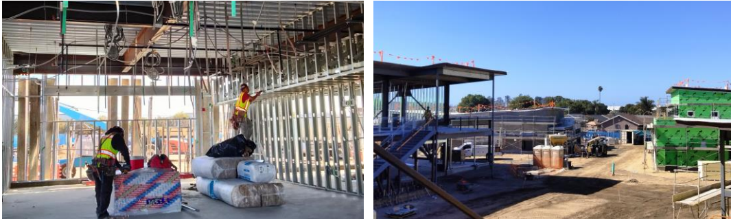
Rose Avenue Elementary School Construction Progress
