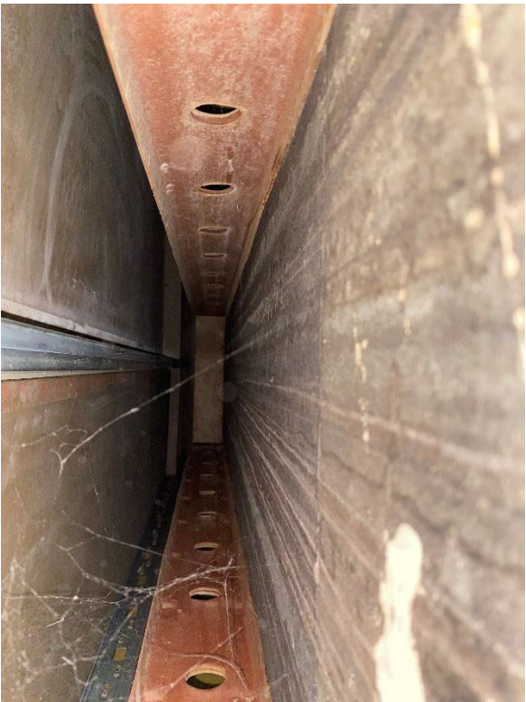
INSUFFICIENTLY STIFF METAL STUD FRAME AND LACK OF INSULATION
