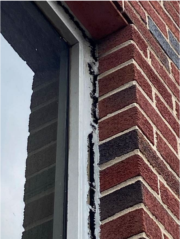
VENEER MOVEMENT AT WINDOW
