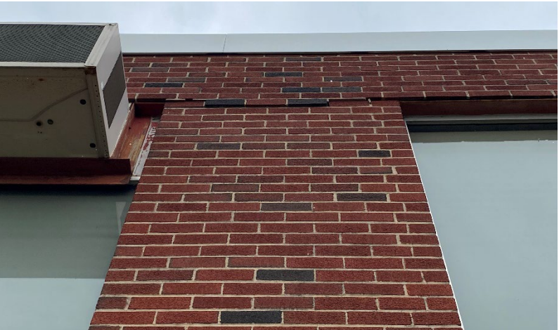
MASONRY VENEER OUT-OF-PLANE MOVEMENT
