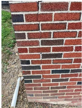
MASONRY VENEER CRACK – EST ELEVATION
