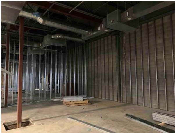
Structural Steel & Metal Framing
