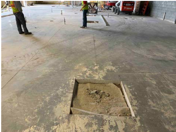
Area B -- Slab Cut New Footings
