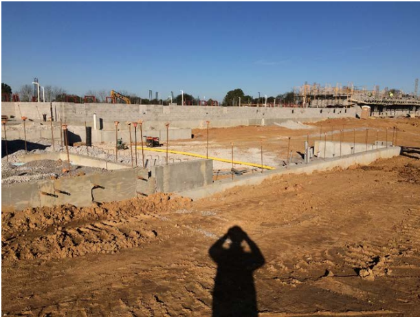
CMU Work (D&E)
