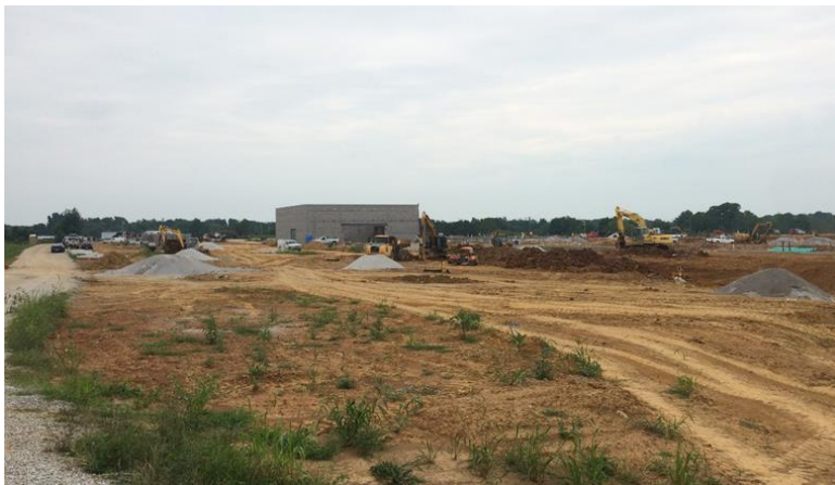
Storm Line Installations
