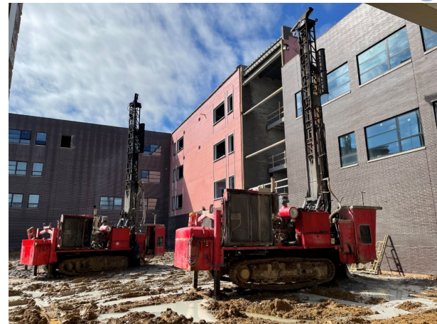
Geothermal Wellfield Drilling
