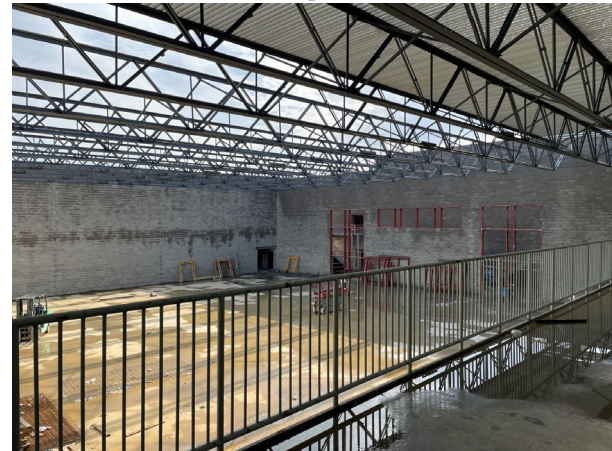
Area F – Main Gym Joists & Deck
