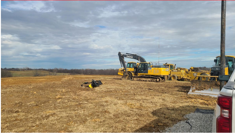
Site Grading at Building Pad
