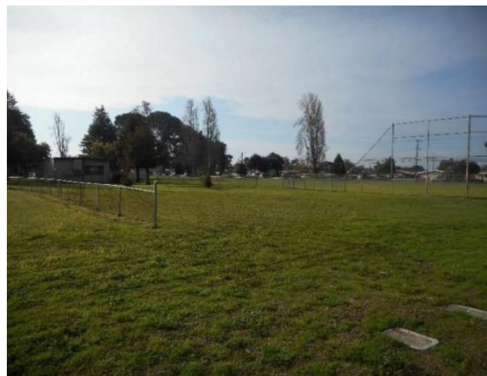
No perimeter fencing at rear of Ruus Elementary School
